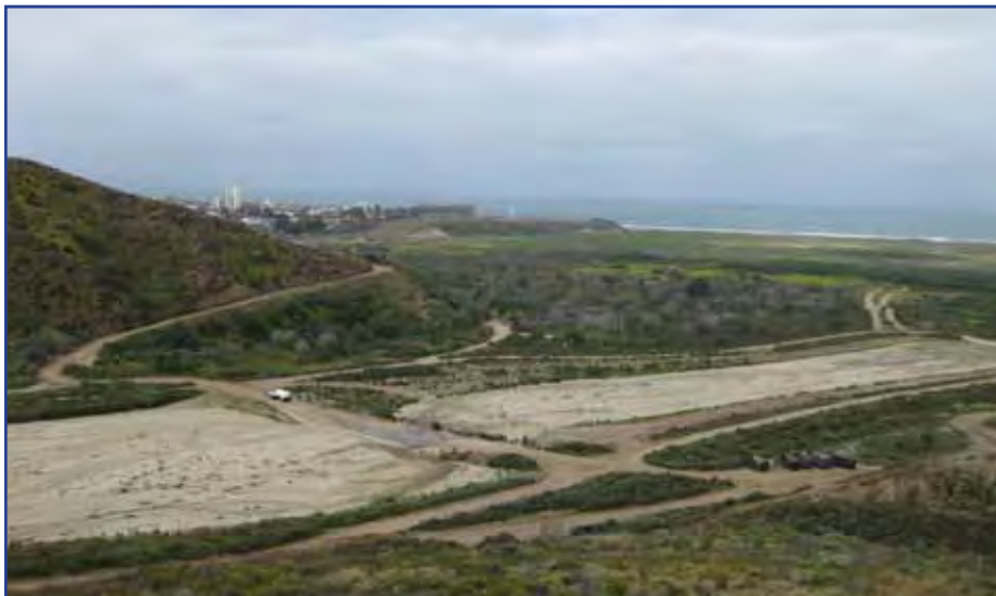
Sediment basins constructed in Goat Canyon capture up to 60,000 cy of sediment from the Cañon de Los Laureles watershed each year
