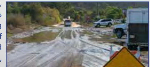
Flooding along Hollister Road in the Valley
