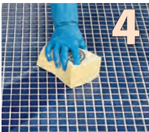
Clean down the tile surface to remove emulsified residues
