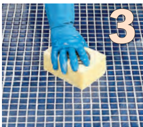
Wash any residue off the face of the tiles when slightly hardened in the joints, and up to 60 minutes after application
