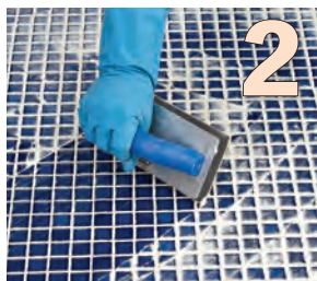
Remove excess ARDEX EG 8 PLUS from the surface
