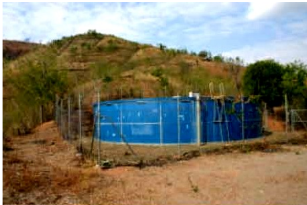
Storage Tank in Dili
