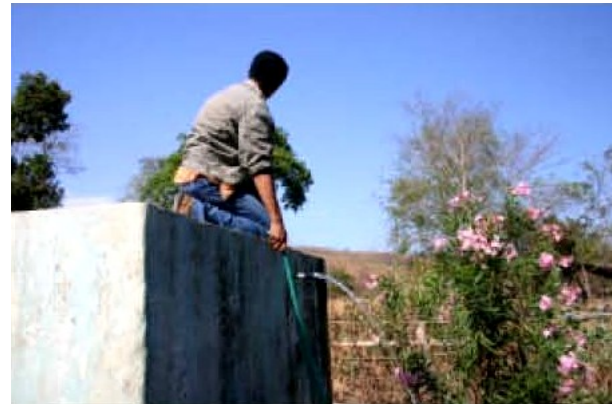
Community-Managed Scheme Illegal Connection from Overflow Pipe
