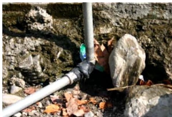
Community-Managed Scheme Control Valve Removed
