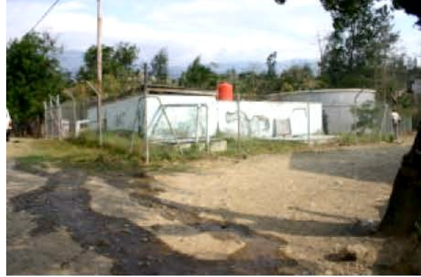
Leaking Storage Tank, Maliana
