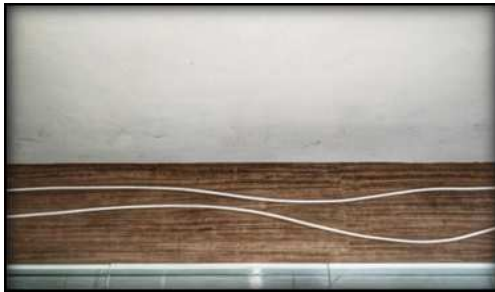
Figure-02: Laid Condition
