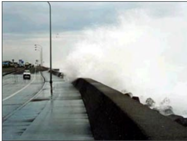
(b) Wave overtopping over the seawall in Hokkaido, Japan
