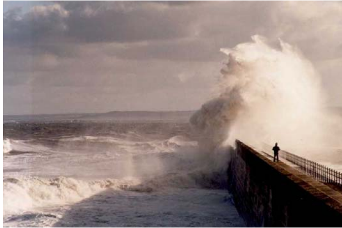
(a) Wave overtopping over the seawall in UK
