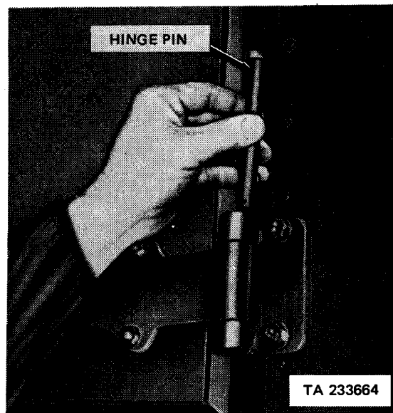
REMOVING OR INSTALLING HINGE PIN
