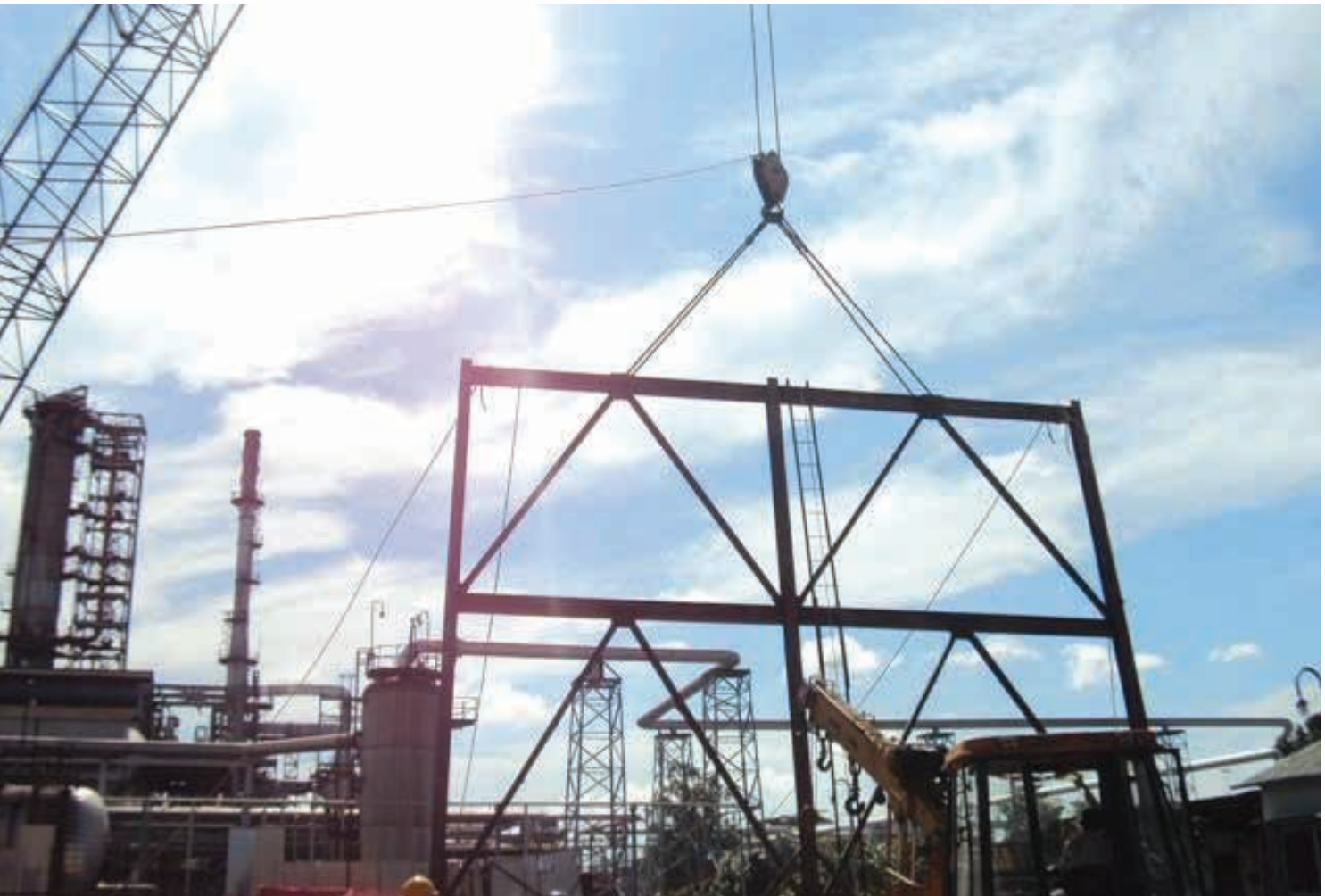
Pipe Rake under erection at Naphtha Splitter Unit
