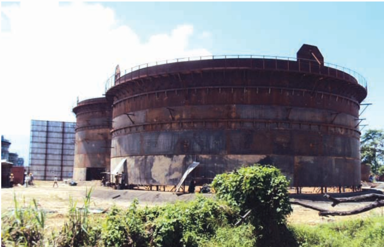
Tankage works under progress at Naphtha Splitter Unit
