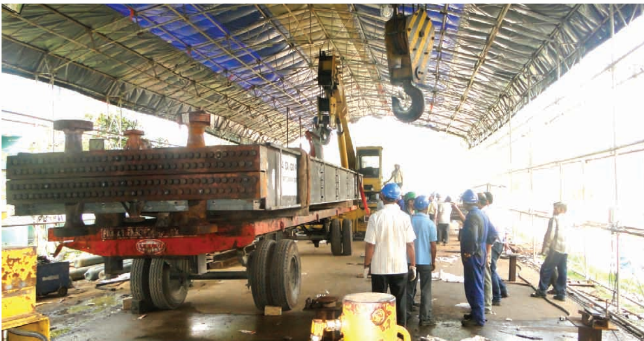
Maintenance work under progress
