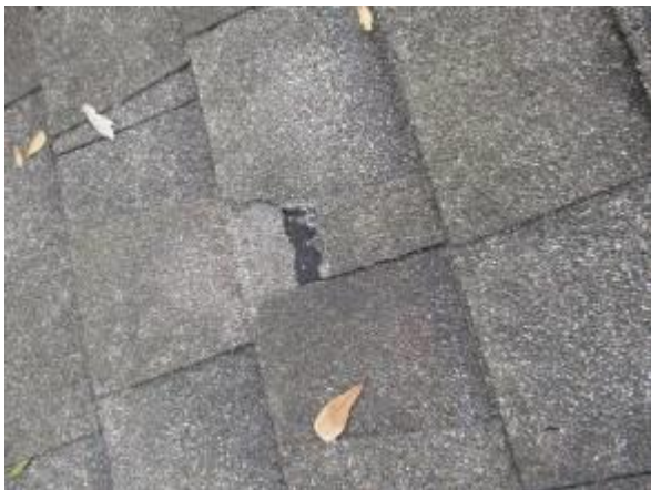
Ivy damaged shingles above the garage
