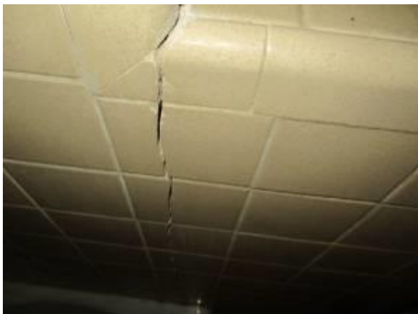
Separated frieze board molding
