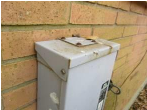
Poor sealant detail
