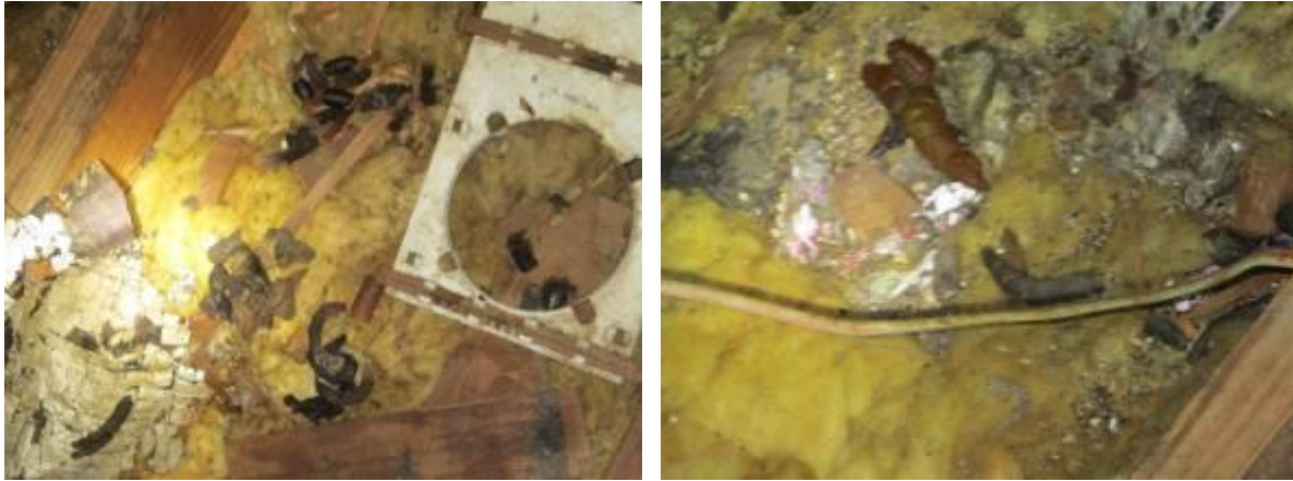
Fresh rodent droppings and a pungent odor were present at the time of inspection
