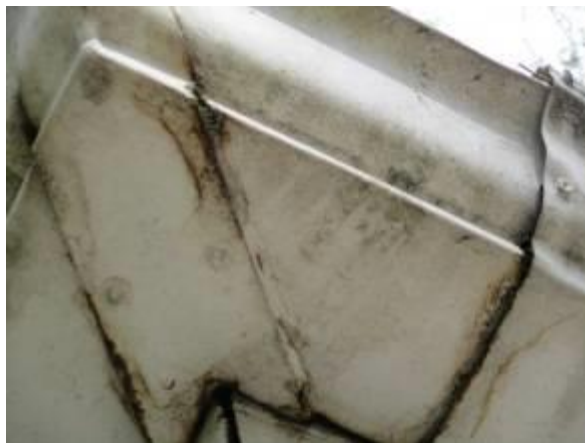
Leaking gutters/Damaged eaves
