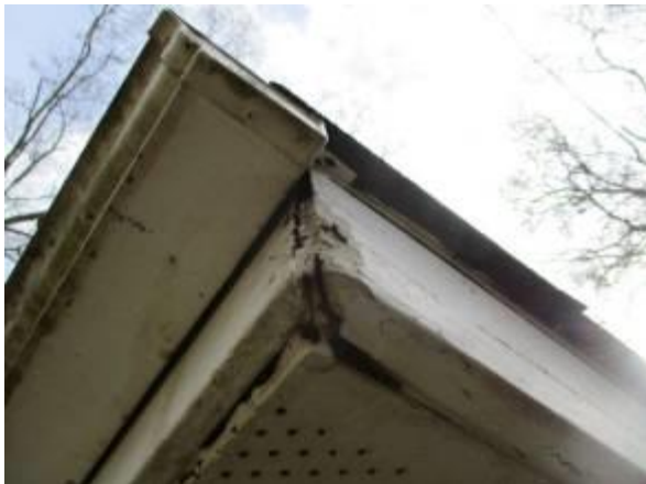
Separated frieze board molding
