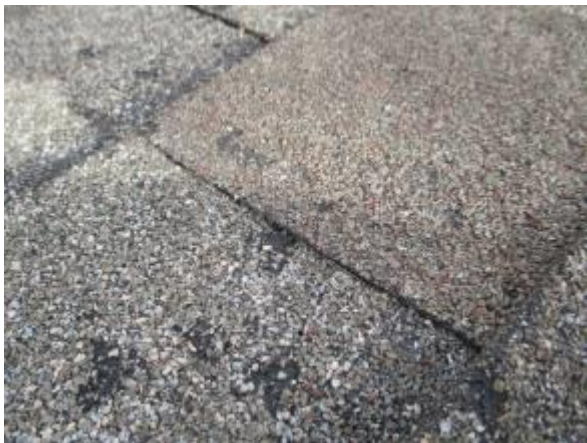
Ivy damaged shingles above the garage
