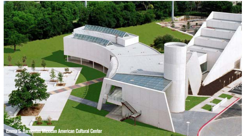
Emma S. Barrientos Mexican American Cultural Center
