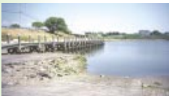
Galilee at Great Island Bridge
