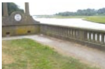
Old Sprague Bridge
