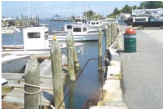
Wickford Municipal Wharf
