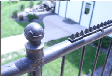
John Barowy helped June 13th fitting loafer rails onto the top of the fencing at the Memorial Community Center.
