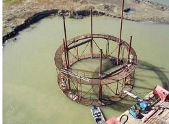
Figure 12 – Installation of wale and strut system and driving the sheet piles
