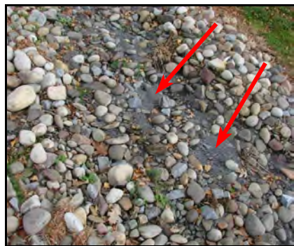
Spaces between gravel clogged with sediment
