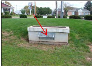
Infiltration basin with infiltration trench extending from spillway
