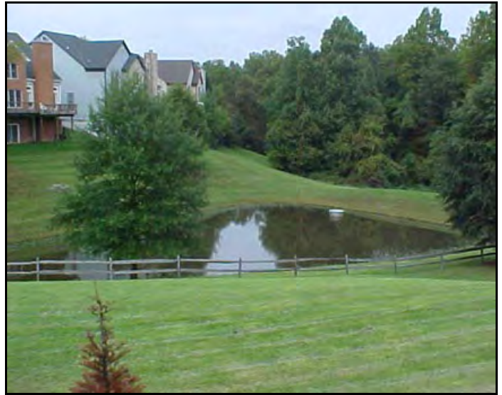
Stormwater Wet Pond from Fairfax County, VA
