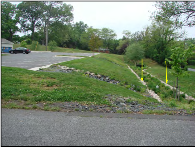
Gravel diaphragm adjoins both sides of bioretention BMP
