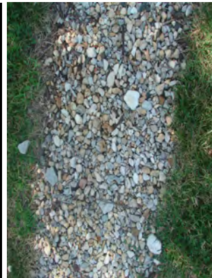
Clean gravel diaphragm
