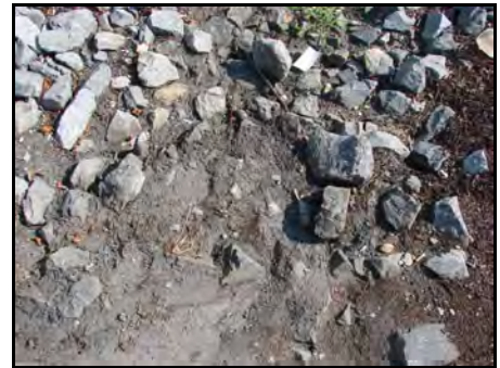
Spaces between stone full of sediment
