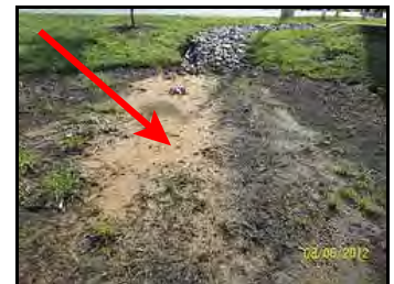
Sediment deposit in BMP
