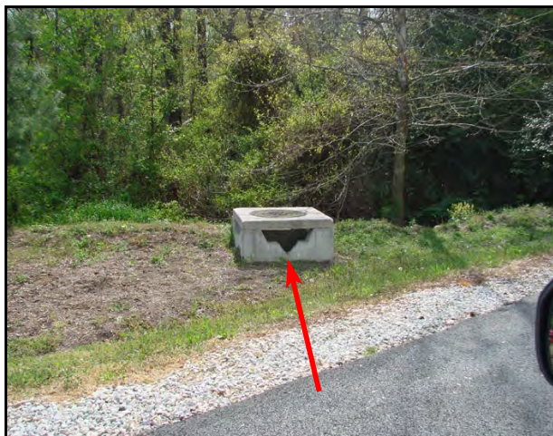
V-Notch cut to prevent ponding
