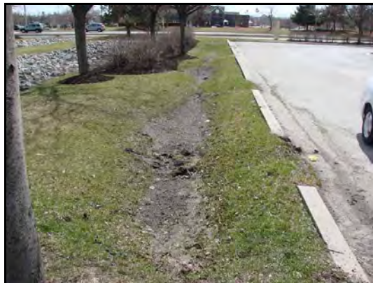
Grass filter strip full of sediment
