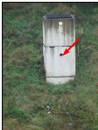
Gravel covers perforated pipe allowing this extended-detention pond to drain completely
