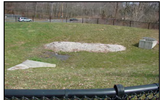
Extended Detention Structure Dry (EDSD) retains runoff up to 72 hrs; Inside gravel dewatering device is a perforated pipe that slows the release of runoff from the pond
