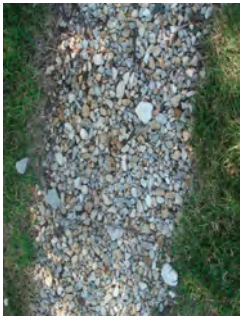
Clean gravel diaphragm
