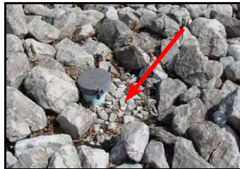
Gravel surface and stone interstices free of sediment
