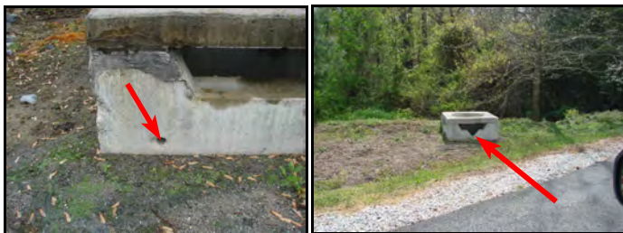
Hole drilled through inlet wall
