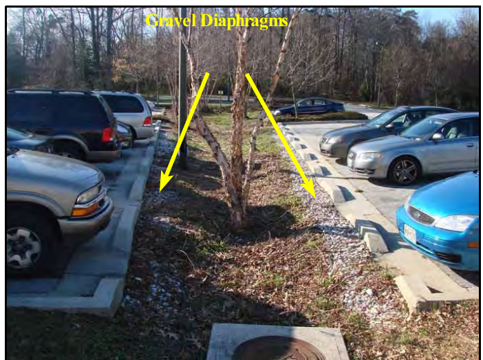
White stone gravel diaphragms along both sides of bioretention
