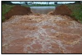
Pond embankment failure from USDA ARS
