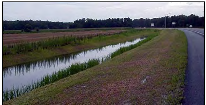
Wet swale along highway in Worcester County, MD
