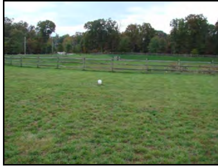
Infiltration Trench beneath lawn; only well visible; can't be assessed
