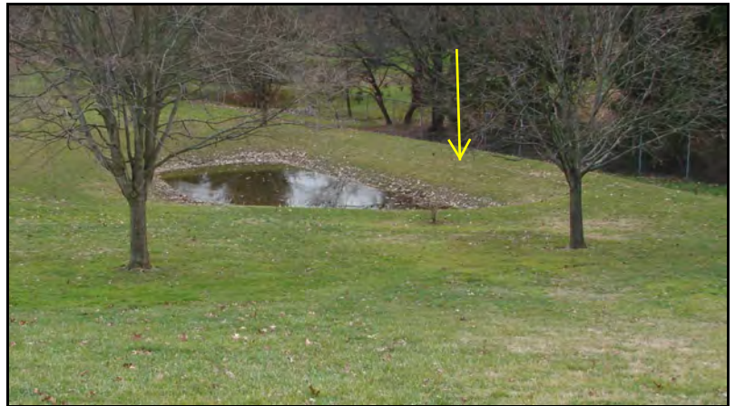
Regular embankment mowing eases assessment
