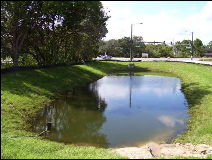
Typical Wet Pond
