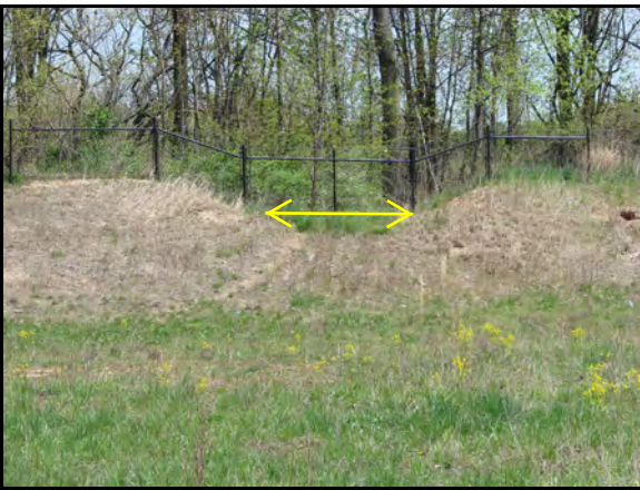
Emergency spillway; an intentional embankment low spot
