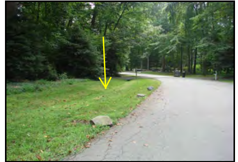
Typical roadside ditch; though runoff from lesser storms infiltrates through ditch bottom a large portion of runoff discharges to a nearby waterway
