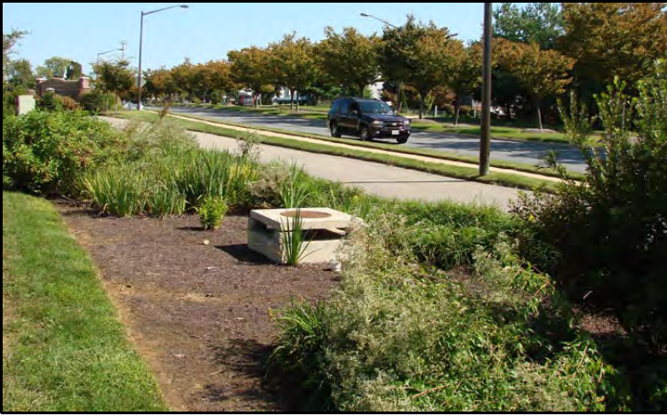
Bioretention (BR) Micro-Bioretention (ESDMB) or Rain Garden (ESDRG): Usually has storm drain inlet with openings one foot above mulched or grass surface; observation well usually present.
