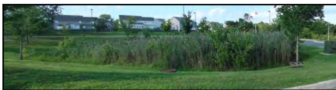
Sand filter overgrown with Phragmites & other wetland plants
