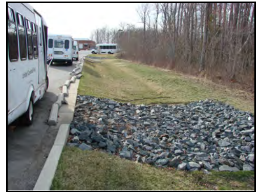
Swale (SW) usually has a wide bottom; observation well maybe present
