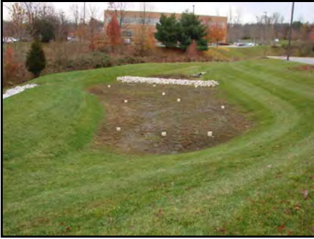
Sand Filter with PVC clean-outs; checkdam forebay for pretreatment
