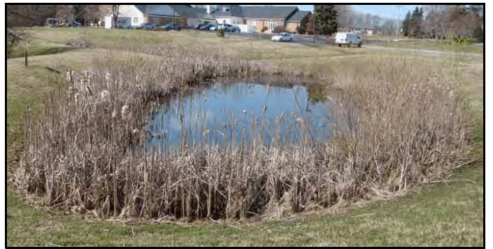
Wet Pond Partially Full With Sediment-Cattails
