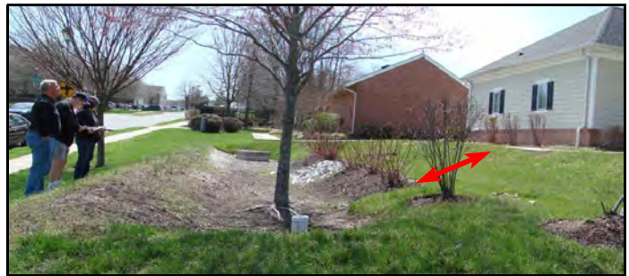
Filter strip between building on right and bioretention center
