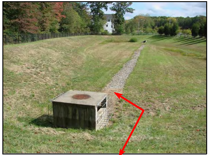
Infiltration basin with infiltration trench extending from spillway
