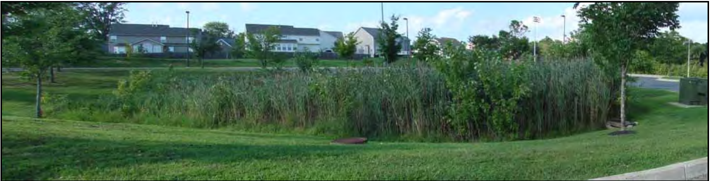
Sand filter overgrown with Phragmites, a wetland plant indicating clogging and that runoff no longer drains completely in 72 hours
