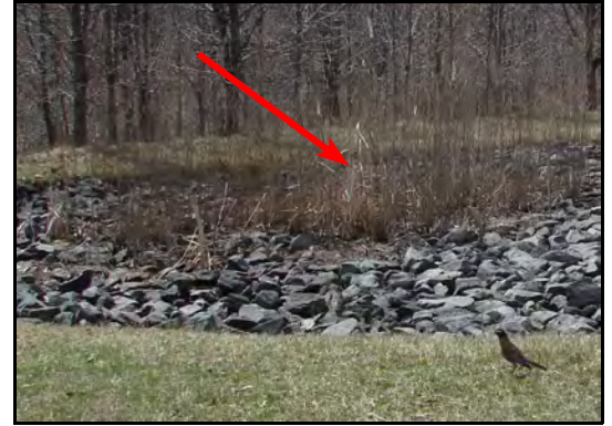
Winter view of cattails in trench indicating runoff no longer infiltrates completely within 48 hours
