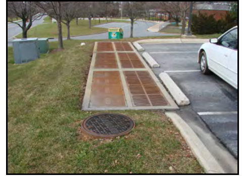
Underground sand filter; very difficult to assess
