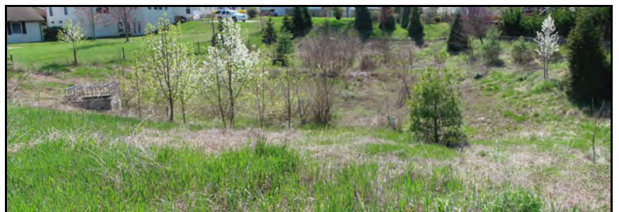
Infiltration Basin overgrown with vegetation
