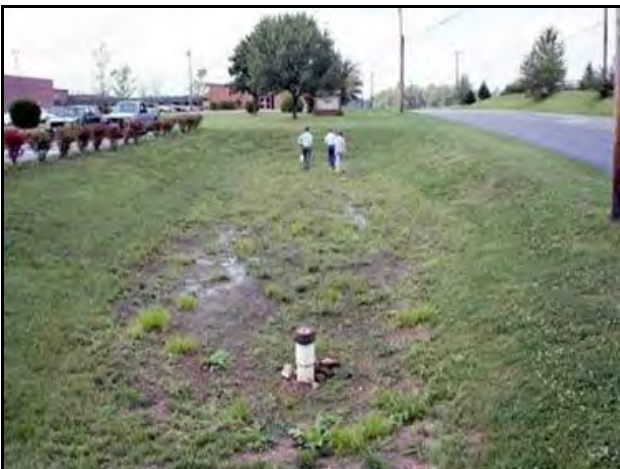
Holding water more than 72 hours after runoff ceases indicates clogging and failure
