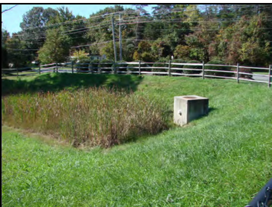
Infiltration Basin full of cattails
