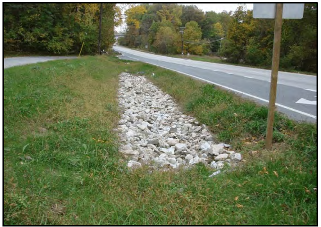
Infiltration Trench With Exposed Stone
