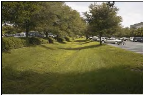
Swale (SW) usually has a wide bottom; observation well maybe present
