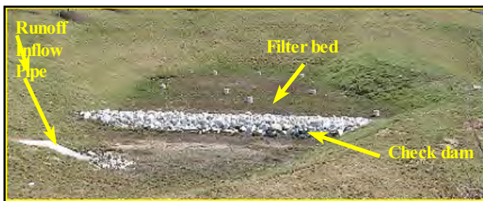
Check dam separating runoff inflow (lower left) from sand filter
