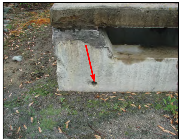
Hole drilled through inlet wall
