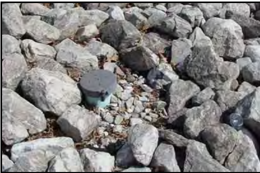
Spaces between stone free of sediment-water
