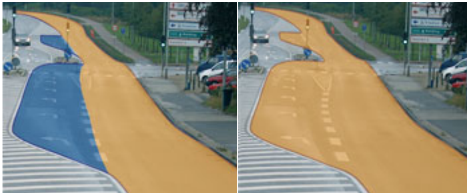
Figure 34: Width controlled spreading from Epoke
