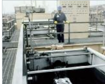
Hydro-Clear® sand filters have proven effective in meeting the stringent discharge requirements of the petroleum industry.
