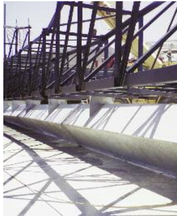
The unitube Tow-Bro® clarifier header, installed at dozens of petroleum refineries and petrochemical plants, ensure uniform and rapid removal of biological solids.
