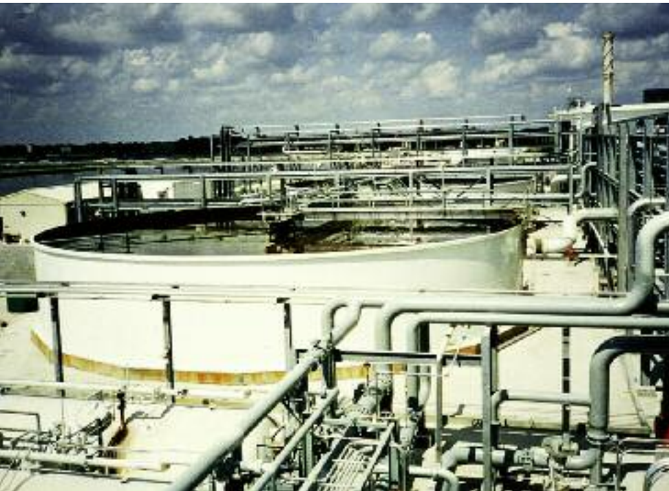
Siemens Water Technologies clarifiers are available in a number of highly efficient and low cost designs, including conventional scraper clarifiers, Tow-Bro® suction clarifiers and Rim-Flo® peripheral feed clarifiers.
