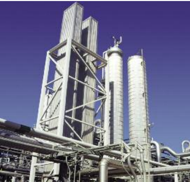
The Zimpro® wet oxidation system is commonly used for treatment of high strength spent caustic generated in petroleum refineries and ethylene plants.
