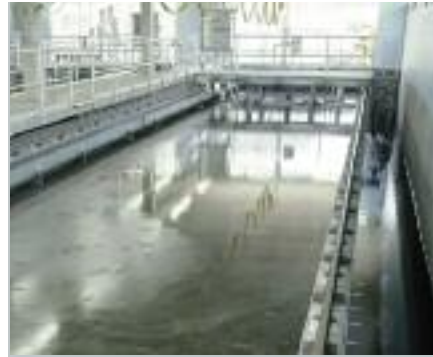
The Gravisand® traveling bridge filter is suited for suspended solids removal and/or turbidity reduction in process water and wastewater.
