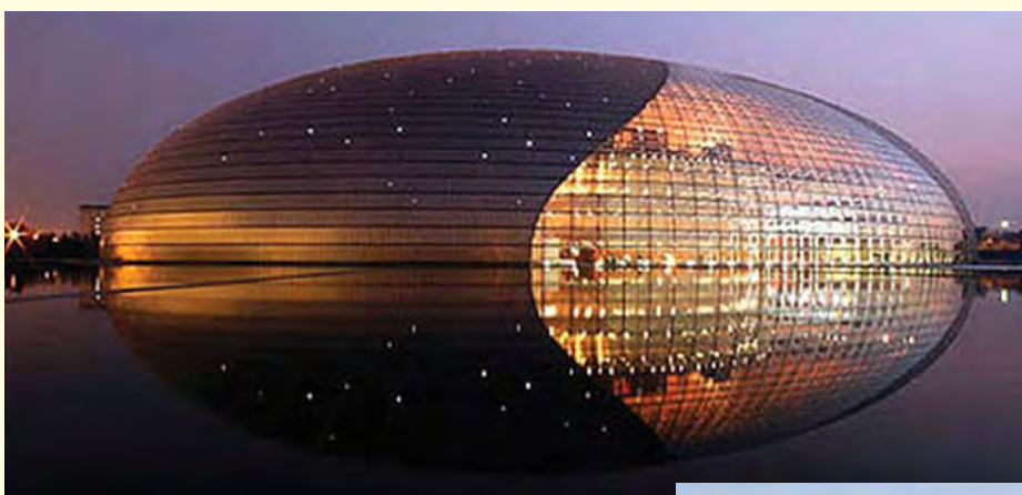
National Centre for the Performing Arts at the Opera House, Beijing.
