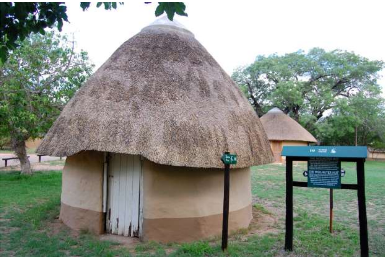
Figure 2: Built in 1930, a surviving example of an early rondavel in Pretoriuskop Camp. These structures were known as “Selby huts” and did not include windows because of the danger posed at night by predators such as lions and leopards Source: Author's own
