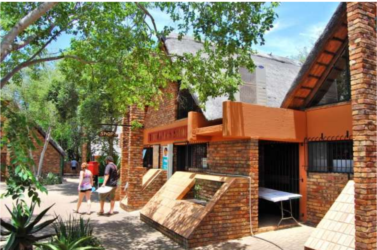
Figure 17: Completed in 1984, Berg-en-dal Rest Camp in the south-western corner of the southern region, represents a departure from the Kruger National Park's traditional architecture style Source: Author's own
