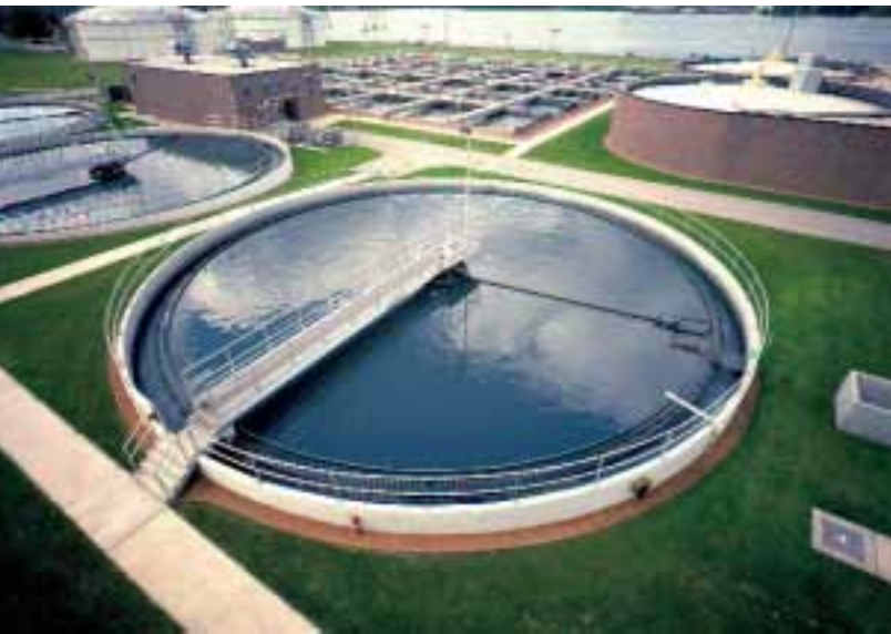
Tow-Bro® for rapid, uniform removal of final clarifier sludges.
