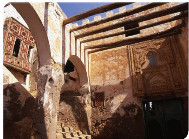
Plate 11 . Inside view of an old building of Suakin in 2007.
