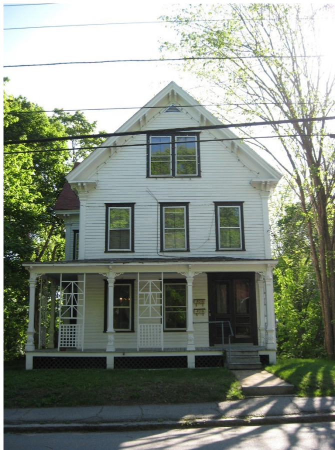
Figure 5. Traditional residential architecture in Spencer..
