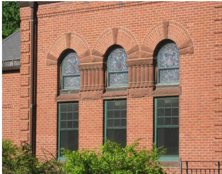
Figure 7. Sugden Library masonry facade.
