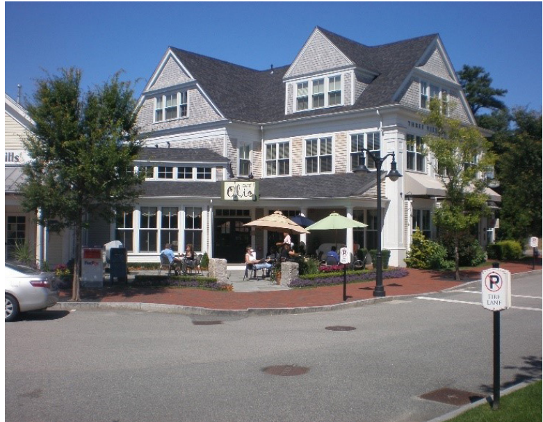
Figure 8. Commercial building in Pine Hills, Plymouth, Mass.
