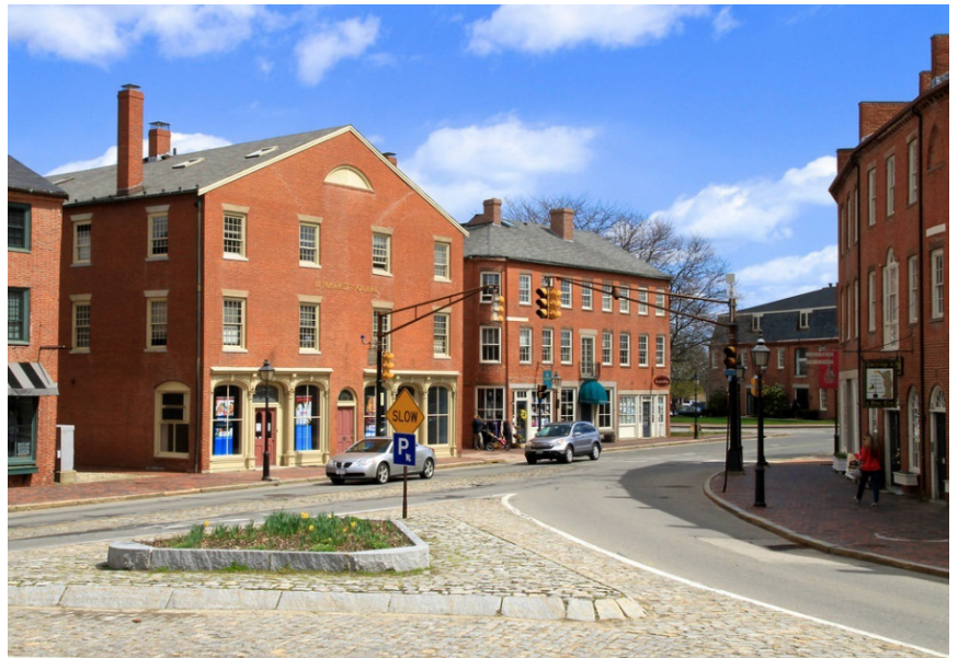
Figure 9. Historic renovation preserving window patterns in Newburyport, Mass (source: Creative Commons).
