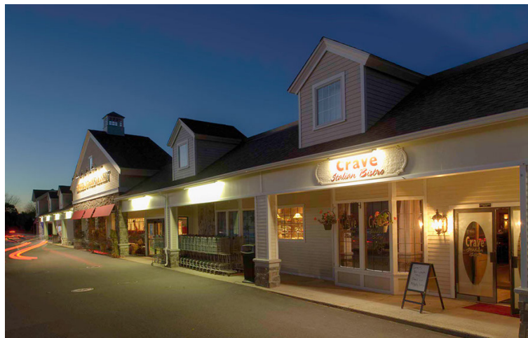
Figure 18. Commercial façade lighting in Southbury Plaza (source: www.tectonarchitects.com ).
