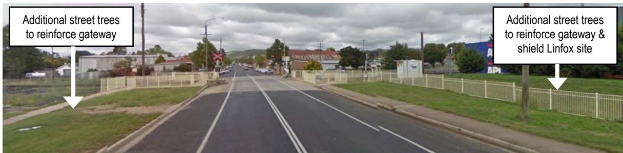
Google Street View: Looking south on Mid Western Highway near railway crossing.
