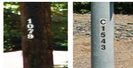
Examples of street light pole numbers
