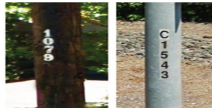
Examples of street light pole numbers
