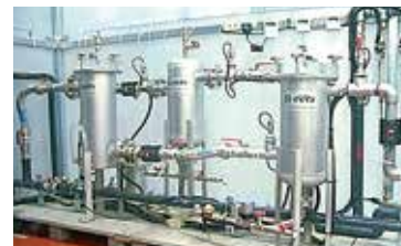
Cooling and circulating water purification systems "Weets"
