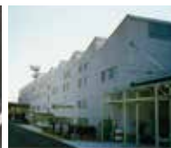
Construction of a filter plant
