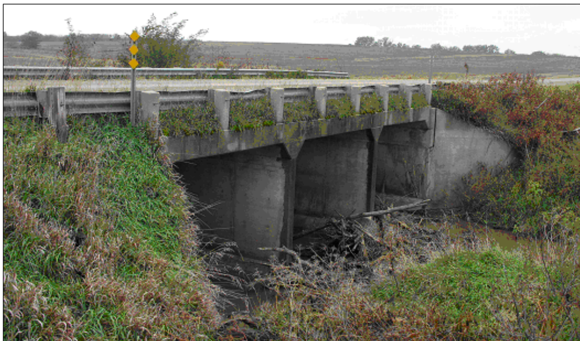
Figure 17. Culvert opening shielded by a guardrail installation
