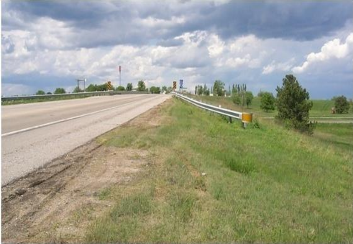
Figure 19. Flared guardrail installation
