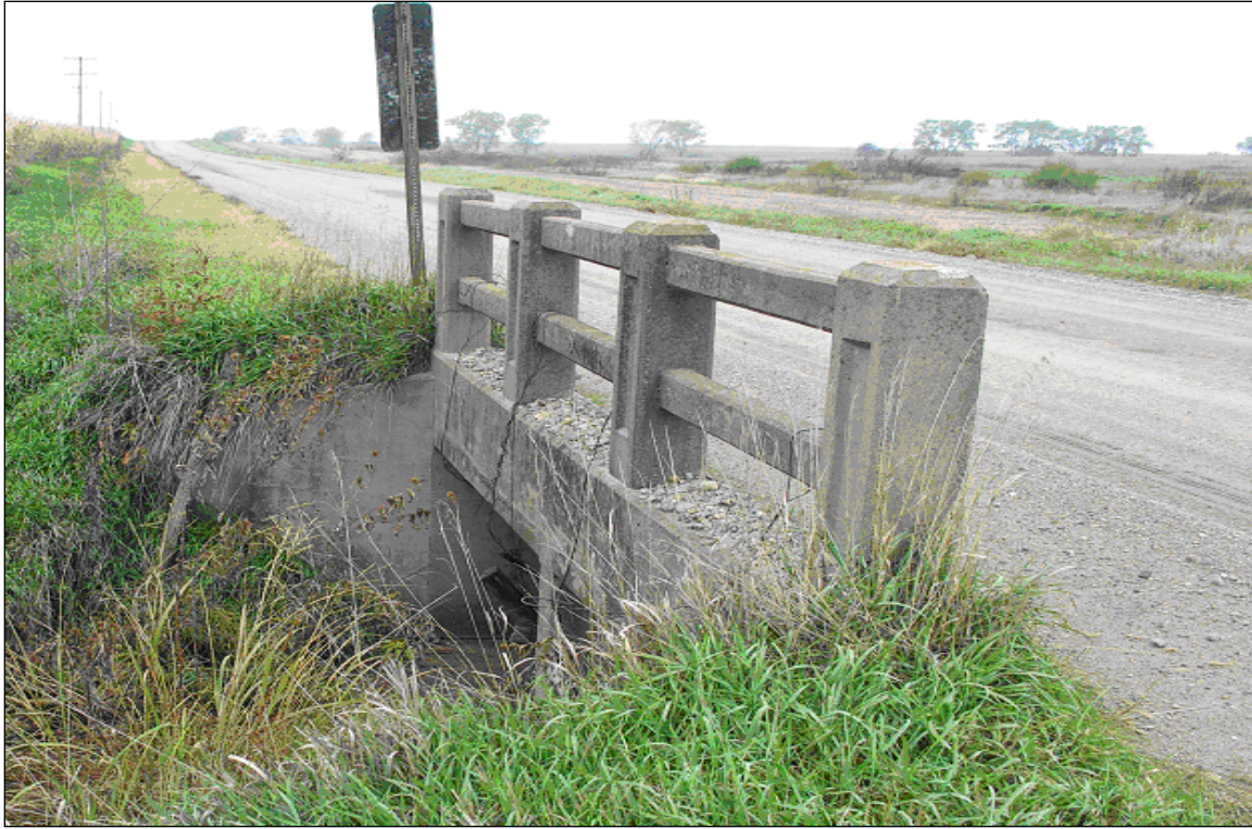
Figure 2. Culvert opening on a local road
