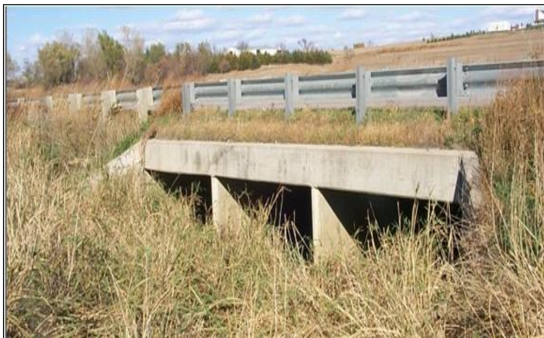
Figure 8. Guardrail installed to shield culvert opening
