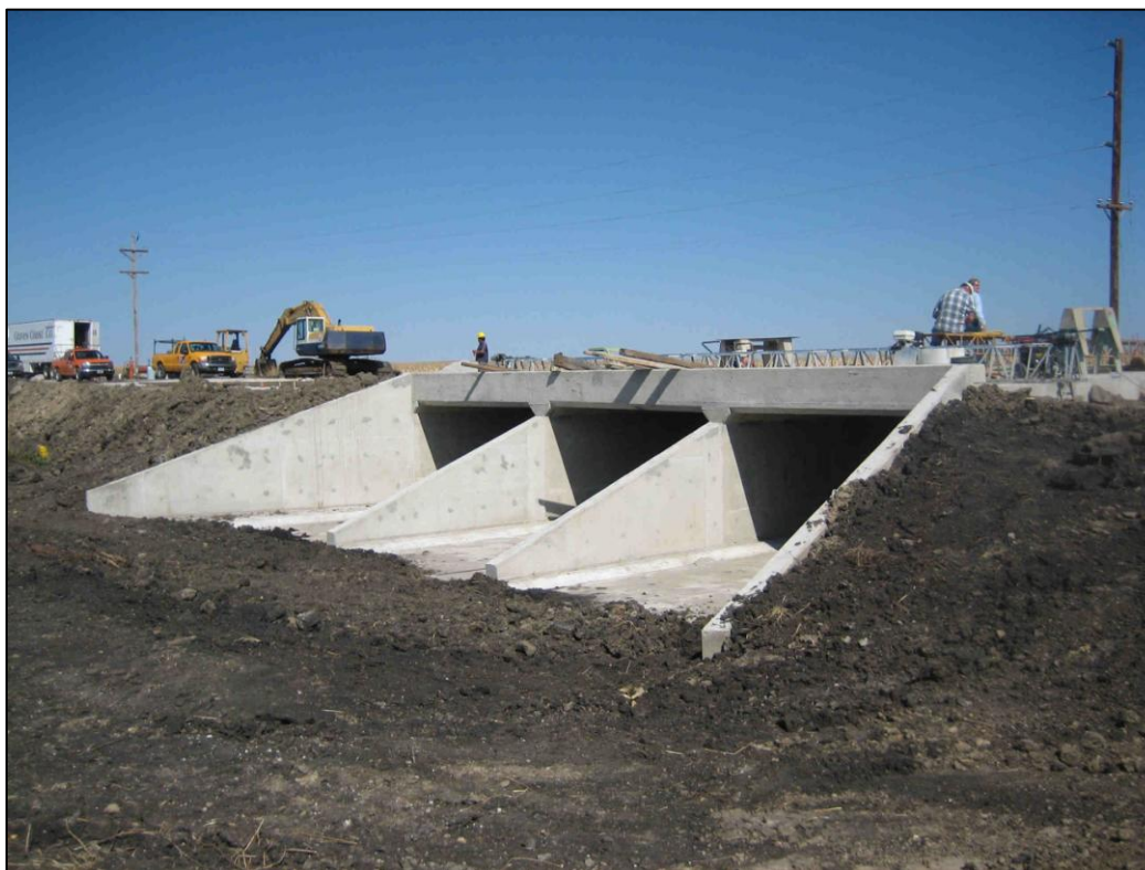
Figure 7. Culvert extension under implementation
