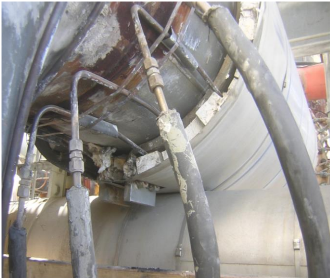
▲ Figure 1. Multiple tracers installed to obtain high heat transfer.
