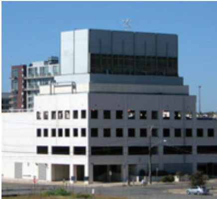
Fig. 3 District cooling tower in downtown Austin, 3rd & San Antonio
