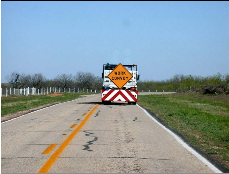
Figure 4. WORK CONVOY Sign on Work Vehicle (TLTW Roadway with Unimproved Shoulders).
