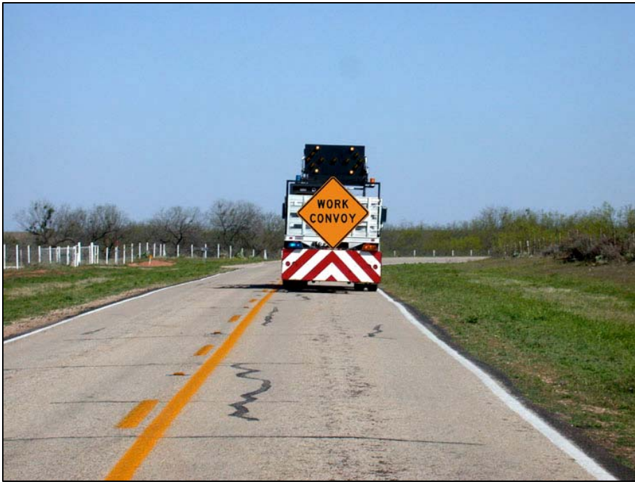
Figure 5. WORK CONVOY Sign and Four-Corner Caution Arrow Panel Display on Work Vehicle (TLTW Roadway with Unimproved Shoulders).
