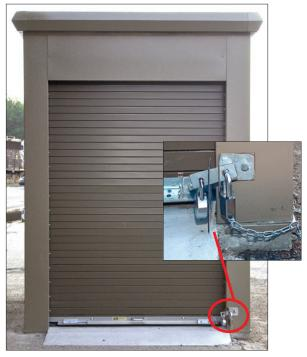
Figure 11-8 – Example of Shed with Locks in the Correct Position
