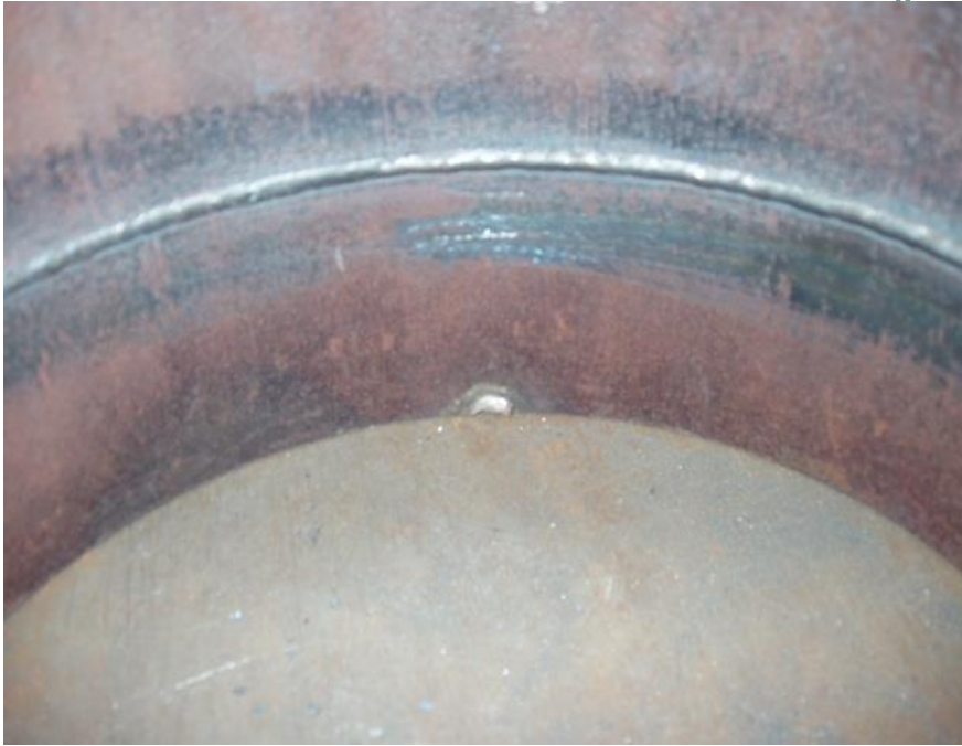
Proper TIG Root weld
