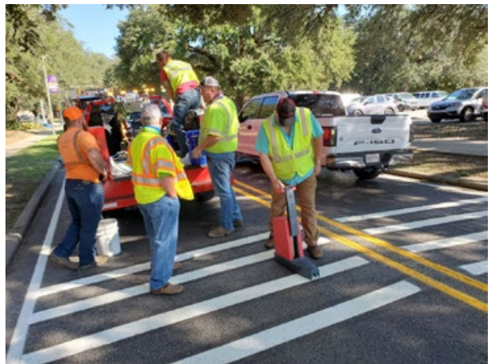
Pavement marking on LSU road.
