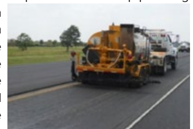
Level-up patching of road at the Concrete Convention and Exposition.
