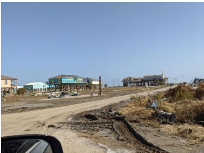
Area in Cameron, Louisiana, affected by Hurricane Laura.
