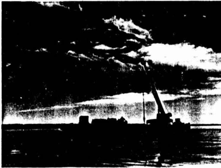
FIGURE 3 40 FOOT X 130 FOOT CRANE BARGE
