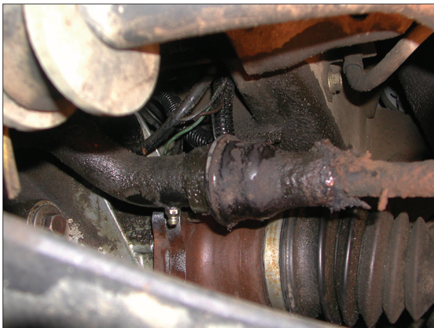
The wiring on this vehicle was damaged but did not actually set a DTC. The code that was stored may or may not have been set by driver operation.
