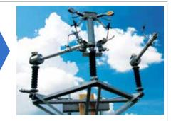
The pick-up finger engages the actuator rod creating a parallel current path. At a pre-determined point, the vacuum contacts separate, interrupting the circuit.
