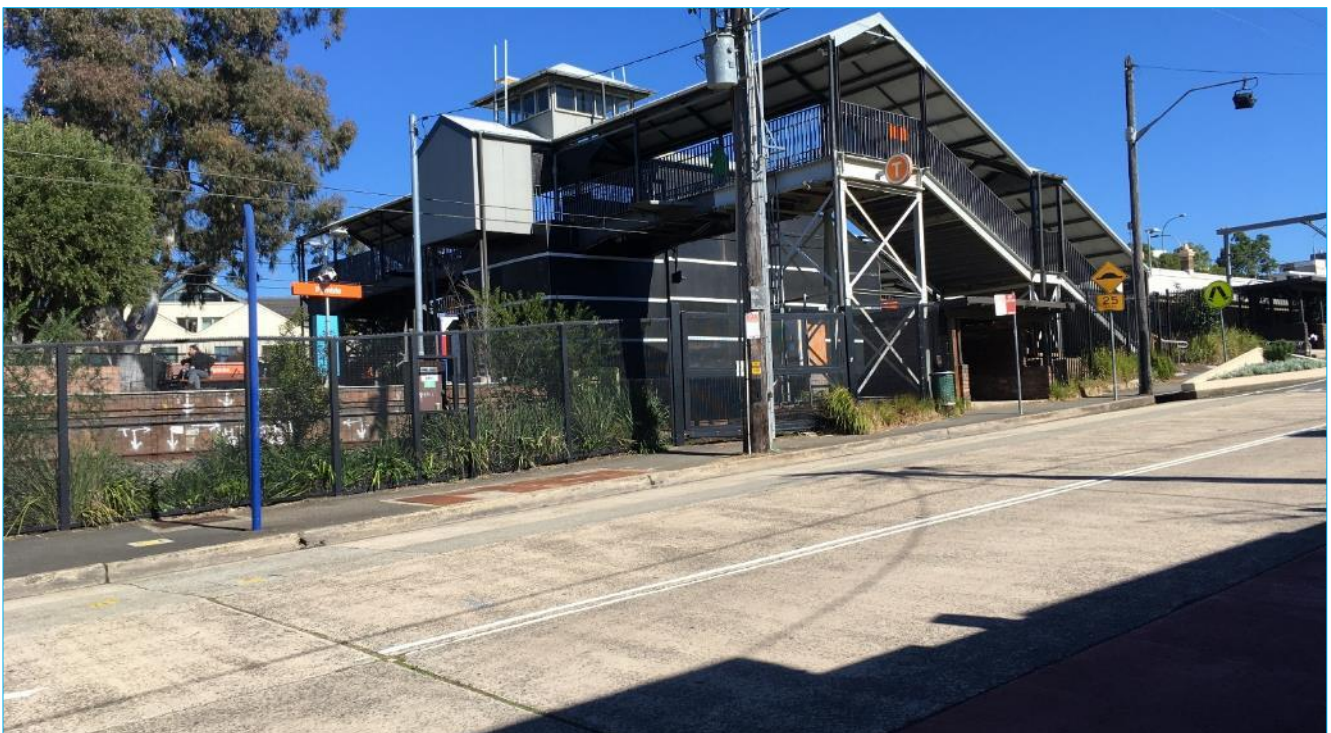
Figure 16: Taxi zone on Grandview Street to the north of Pymble Station
