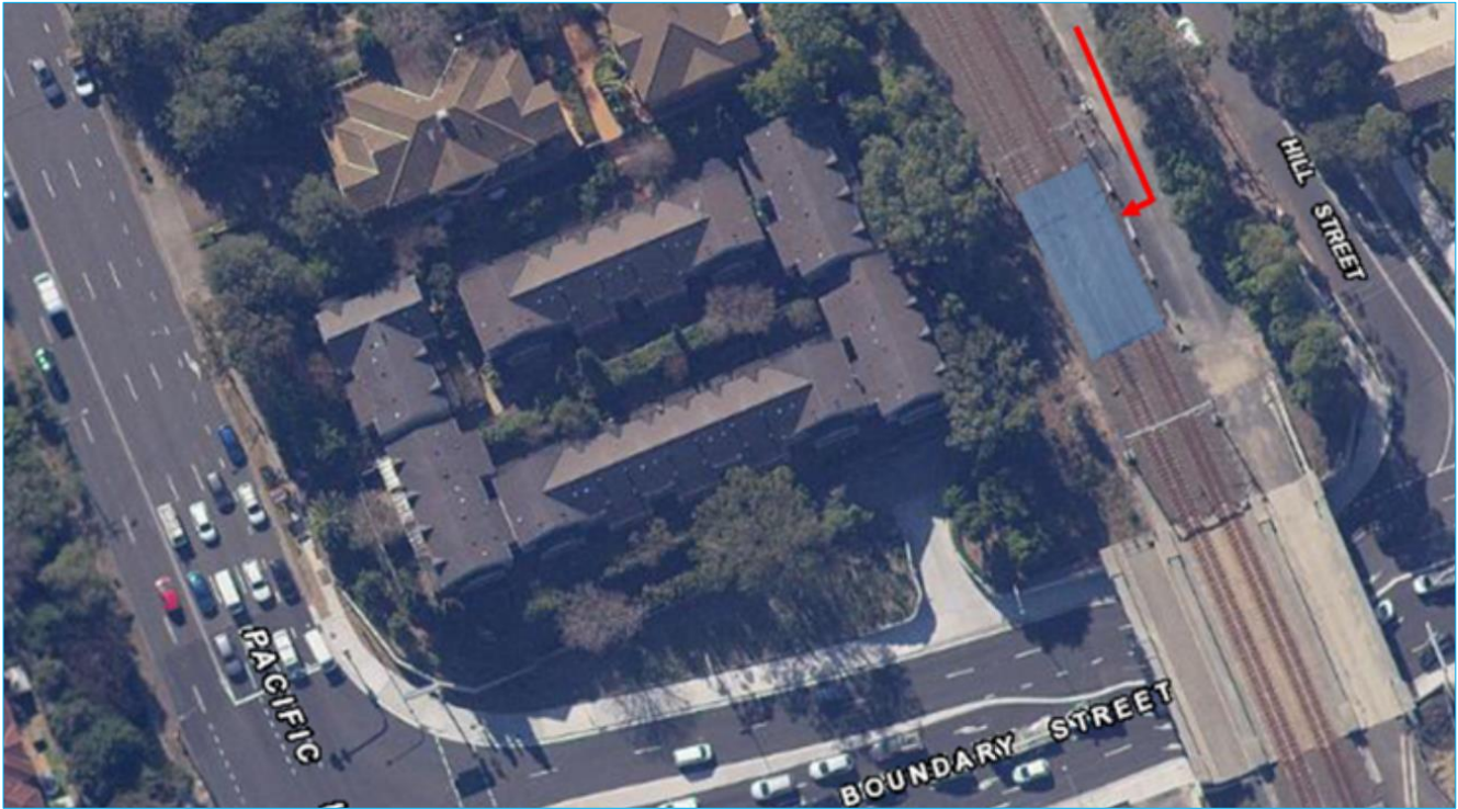
Figure 32: Hi-Rail Vehicle Access to Rail Tracks via Hill Street, Roseville
