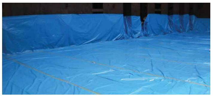
Figure 3.9 | Kraft paper overlaid with plastic sheeting on the tank top and continue vertically along the corrugated transverse bulkhead.
