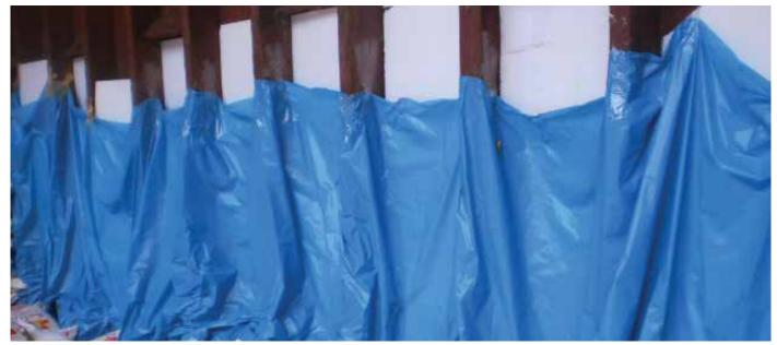
Figure 3.7 | Styrofoam laid between sideshell frames and then overlaid with blue plastic sheeting.
