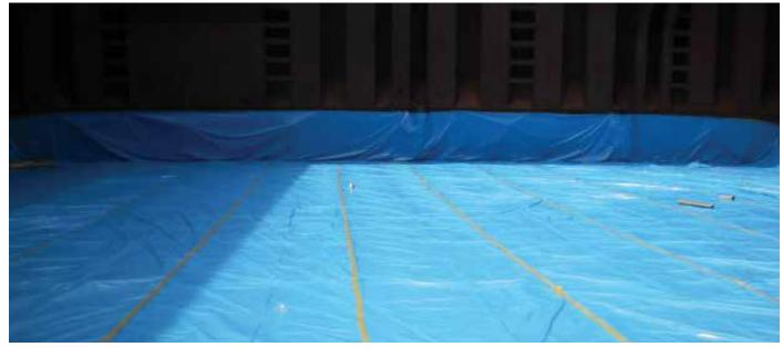
**Figure 3.6 I** Kraft paper overlaid with plastic sheeting on the tank top. This continued vertically along the corrugated transverse bulkhead in background.
