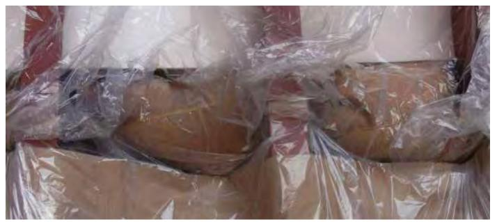
**Figure 3.17 I** Saw dust in burlap bags is inserted at transition point between sideshell and top of hopper tank. Notice the Styrofoam sheets above and kraft paper beneath the bags is then overlaid with plastic sheeting.
