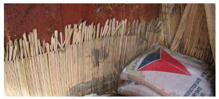
**Figure 1.6** I Bamboo mat dunnage along the ship sideshell has been stained through ship sweat. The bag adjacent to the dunnage has been stained through the migration of condensation though the bamboo mat into the bag.
