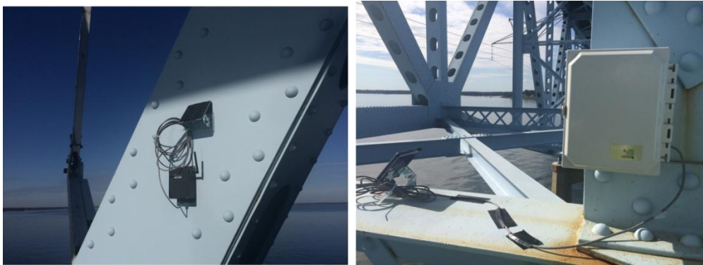
Figure 9: Installation of Solar Powered SeniMax Gateway and Repeaters installed on Bridges
