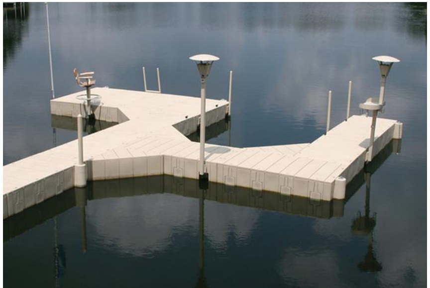
Figure 4.12 Dock Installed by Northwood Dock and Service
