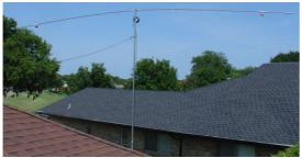
Photo E: Completed 17/12M trap dipole
