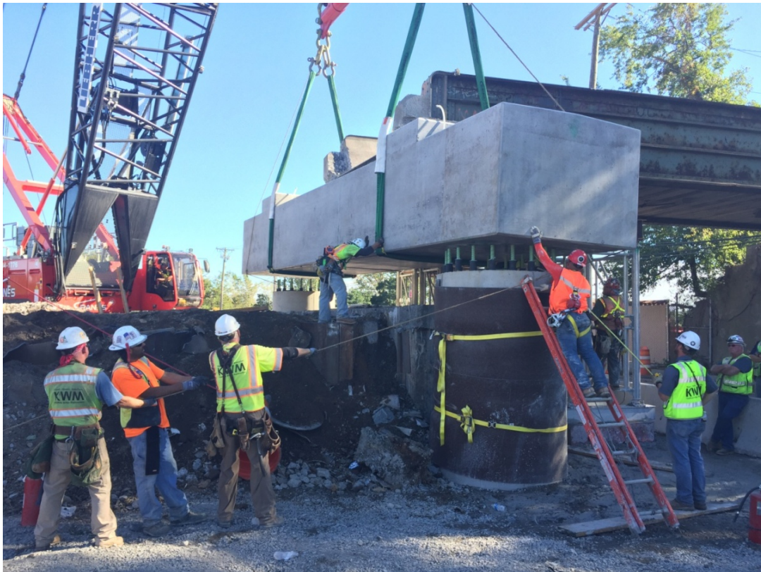
Photograph 1. South Pier Cap Erection
