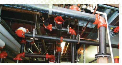
**HVAC HEATING SYSTEM** Two variable speed heating pumps were installed for more efficient operation. The piping system of the existing boilers was modified to achieve variable hot water flow. The entire perimeter radiation system was removed as a result of the increased performance of the building envelope.
