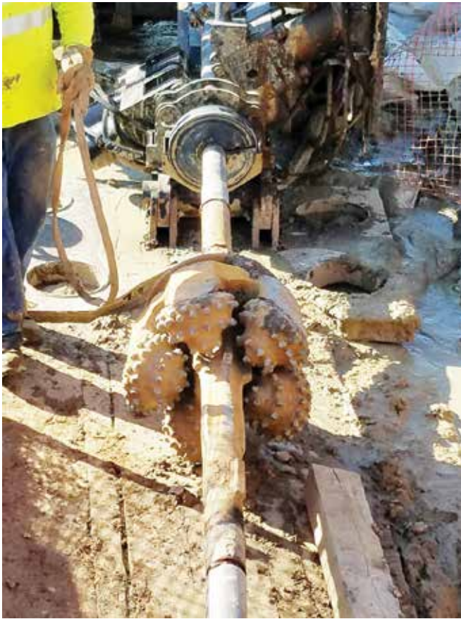
Thorough geotechnical investigations should be conducted before construction in all areas of planned HDD activity
