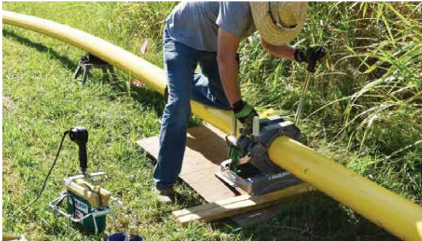
Joining PA 12 pipe is easy and fast, saving time and money
