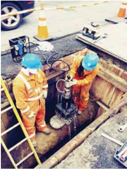
Crew preparing main for CISBOT
