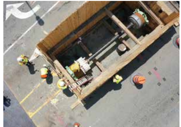
Receiving pit, Central Avenue West
