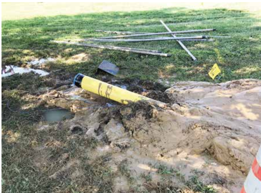
Lack of corrosion concerns dramatically reduces ongoing maintenance
