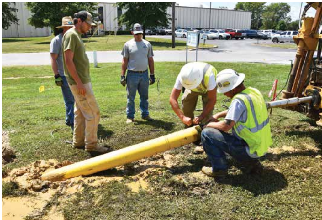
Hard smooth coated surface of PA 12 helps pullback
