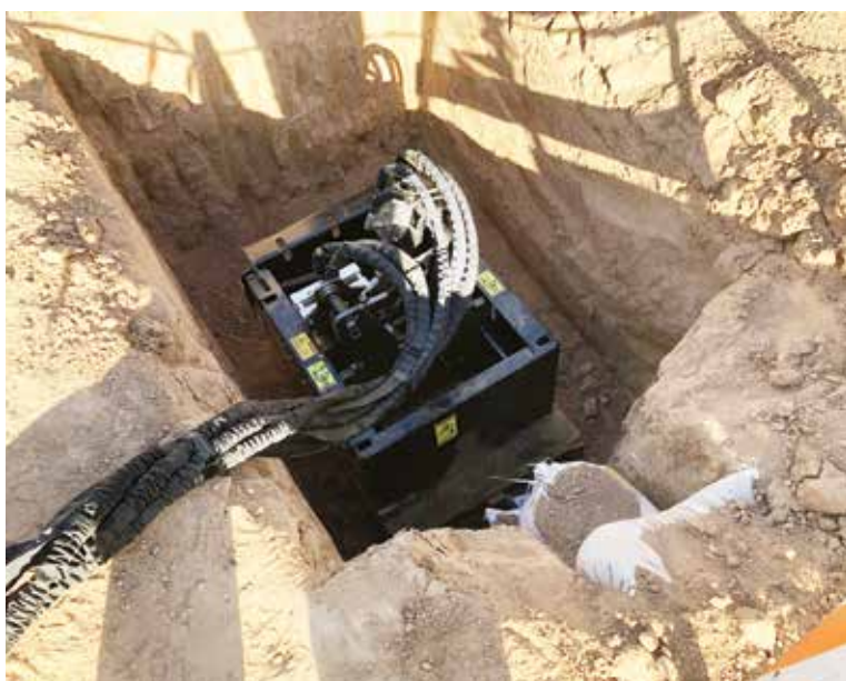
The pipe extractor requires a small excavation to access the pipe to be replaced. Minimum machine pit size is approx. 30 x 27 inches
