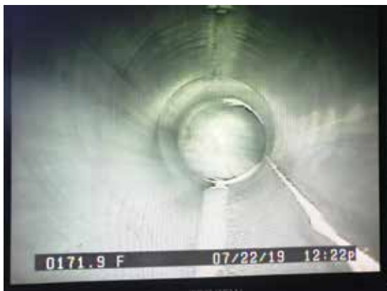
Final post-lining CCTV
