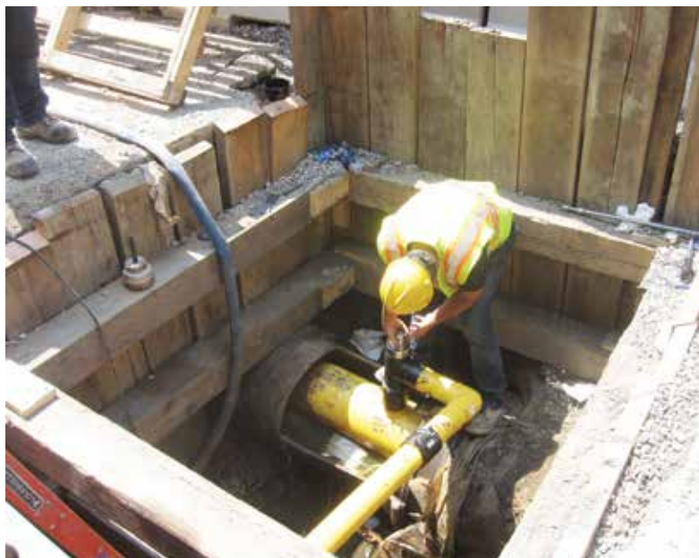
Figure 7 – Site 1: New Service for Large Residential Development
