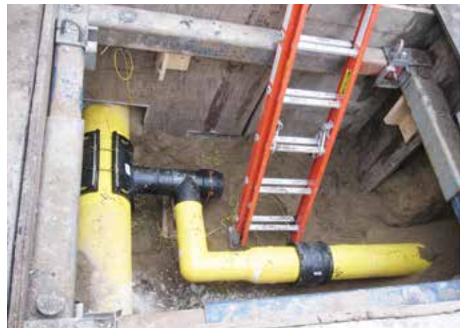
Figure 2 - Supraflow Excavation Pit
