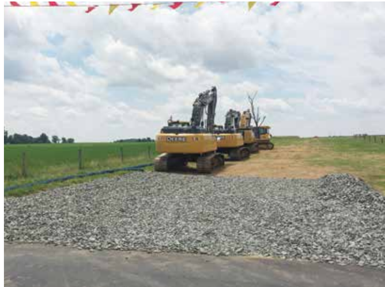
Important to maintain clean and orderly project access points
