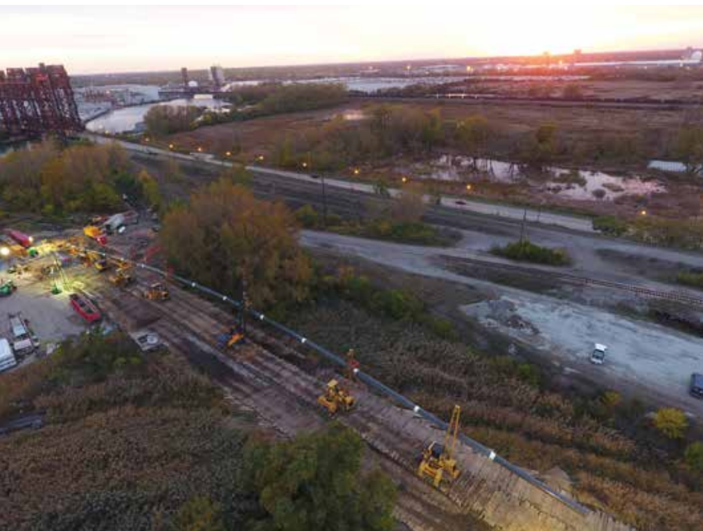
Record-setting 36-inch direct pipe installation 30 feet under the Calumet River
