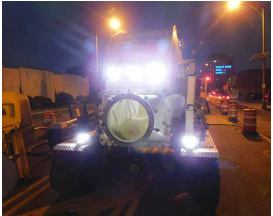
Because of summer heat-wave, work began at 4am installation day
