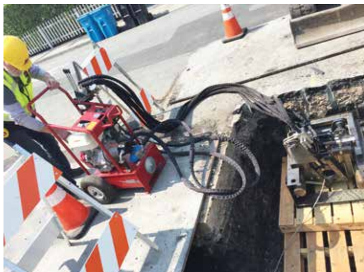
The hydraulically powered extraction machine generates up to 13.3 tons of pulling force and is operated from outside the machine pit
