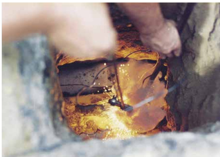
Attaching anode for cathodic protection to steel gas line using cad welding
