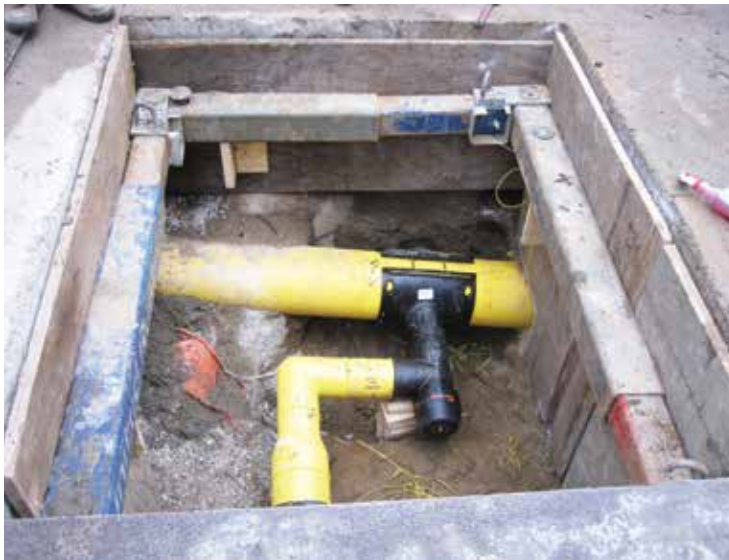
Figure 9 – Site 3: Horizontal Service Installed on an Inclined Main
