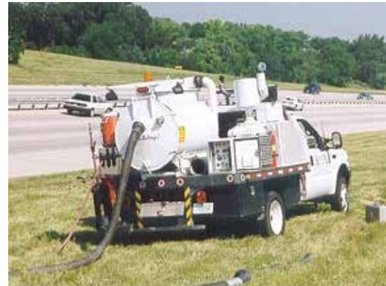
Vacuum potholing, or “daylighting”, continues to be the definitive method
