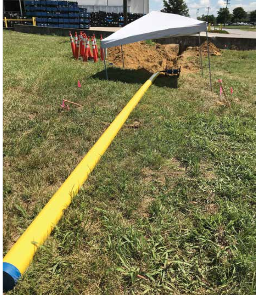
More ductile and lighter than steel pipe, PA 12 is easy to install
