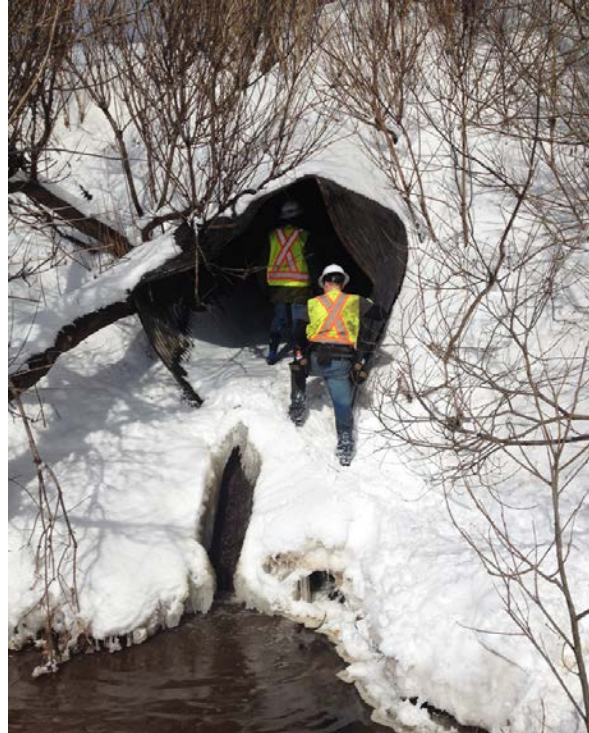
Figure 11. Outlet of pipe.
