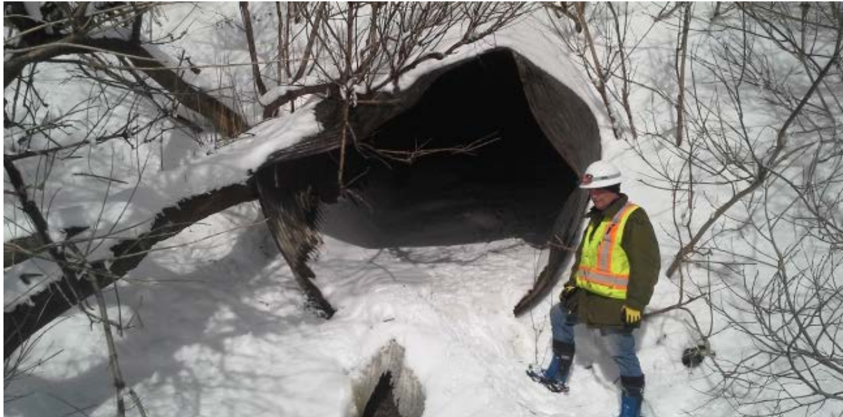
Figure 13. The outlet of the CMP asset.
