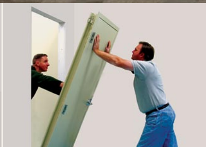
Set assembly in opening.
