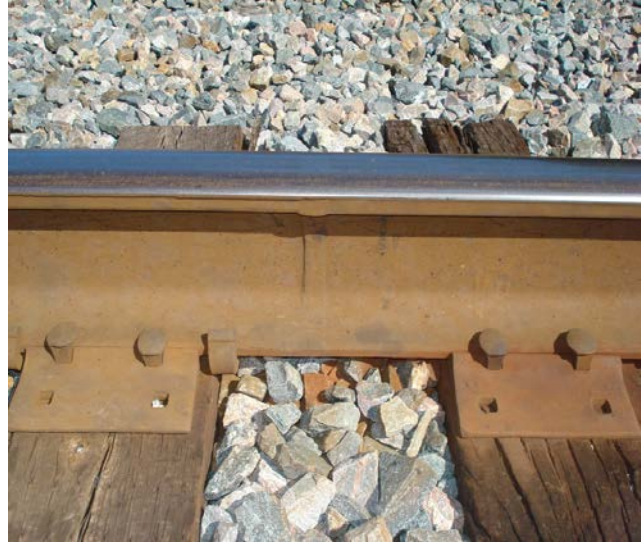
Figure 54: Electric Flash Butt Weld in Track
