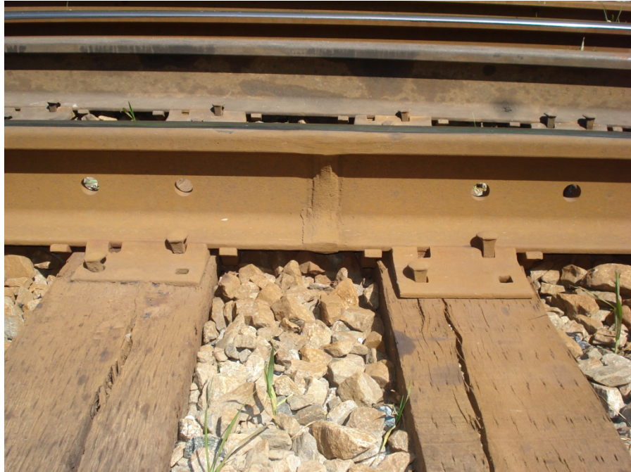
Figure 57: Thermite Weld in Track
