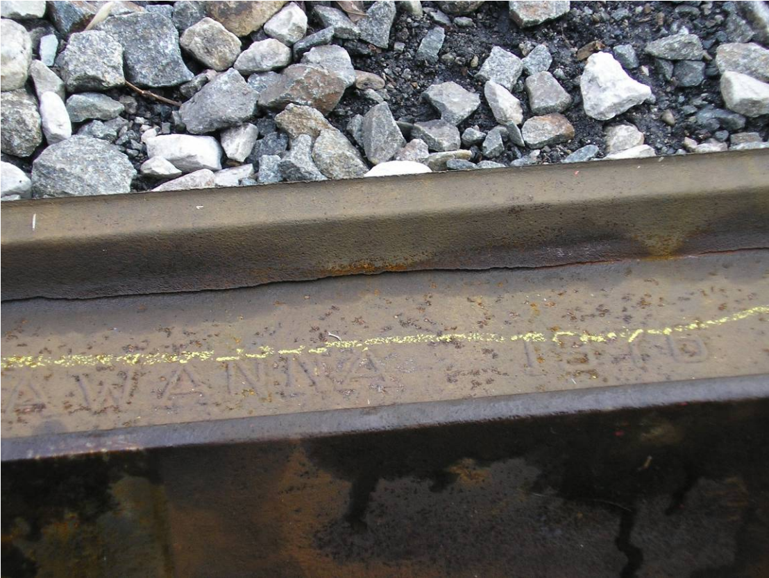
Figure 25: Vertical Split Head Crack Out in Head/Web Fillet Area
