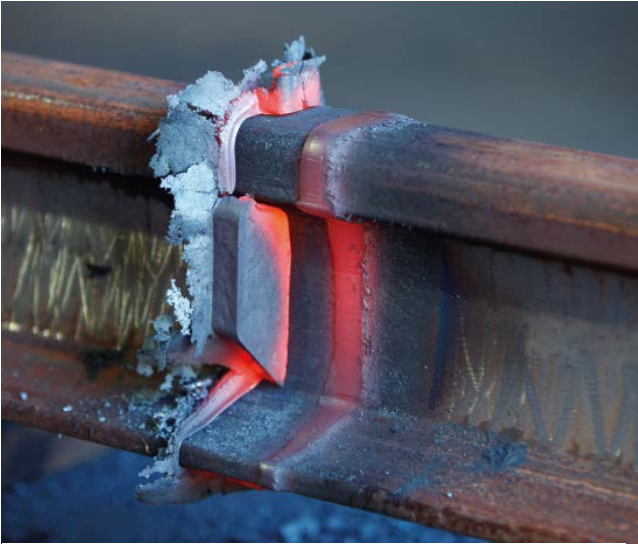
Figure 53: Newly Completed Electric Flash Butt Weld
