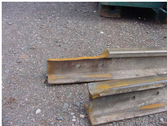
Figure 29: Head and Web Defect Associated with Rail Joint
