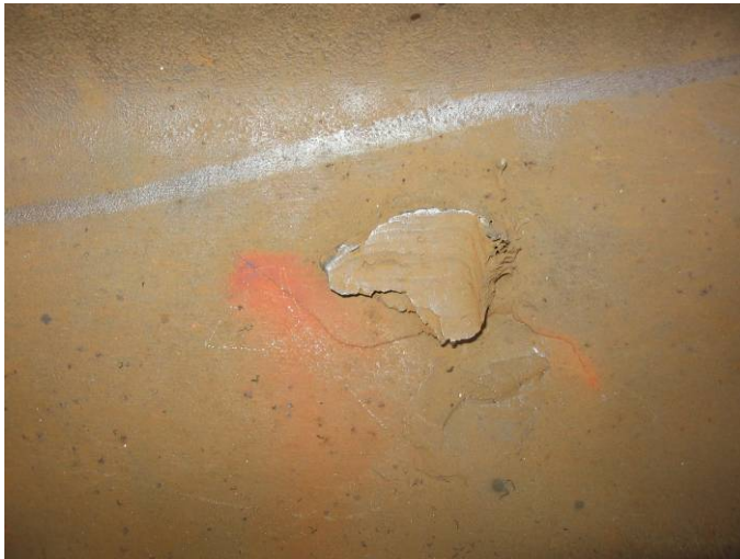
Figure 42: Web Defect Developing from Bond Application
