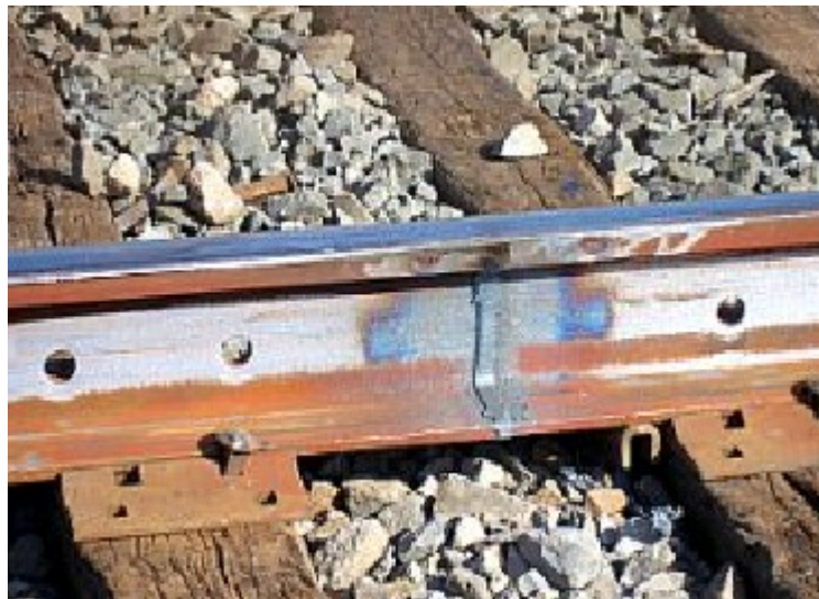
Figure 55: New in Track Electric Flash Butt Weld
