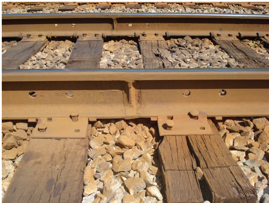
Figure 58: Boutet Weld in Track
