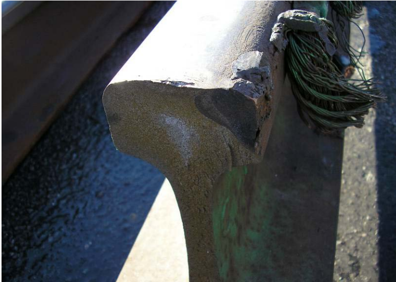
Figure 41: Transverse Defect Developing from Bond Application
