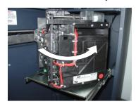
Figure 4-15. Rotate mechanism to operate position (counterclockwise).
