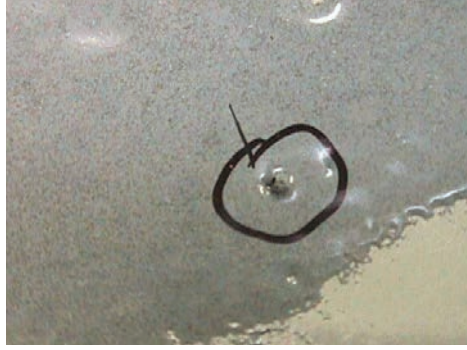
Img. 3.5.2. Surface defect caused by a foreign body
