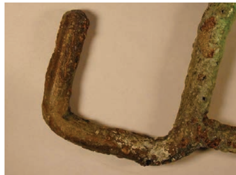
Img. 2.3.2. No earthing at multi coated hooks
