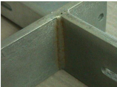
Img. 3.9.1. Insufficient wet out caused by corrosion
