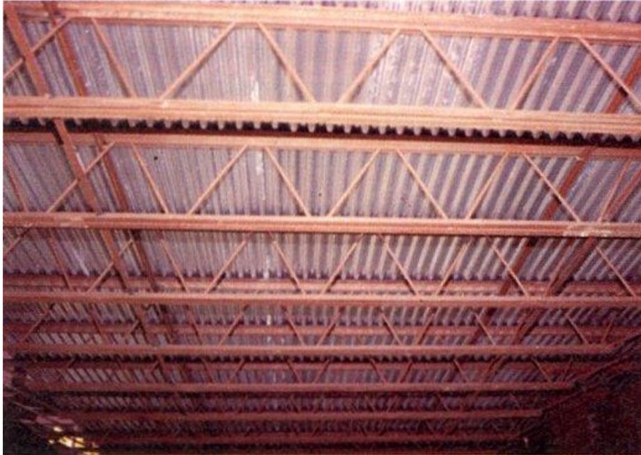
Figure 64: Open web bar joists.
