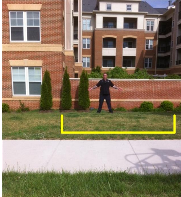
Figure 19: The area where this firefighter is standing is actually designed for fire department vehicle access. The compacted soil and tile blocks are hidden beneath the grass. These kinds of hidden vehicle access points need to be readily displayed on maps and preplans.
