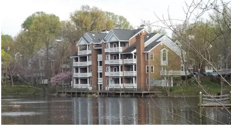
Figure 6: Obstacles like waterways can drastically affect truck company positioning. When discovered, these obstacles must be reported the command post.
