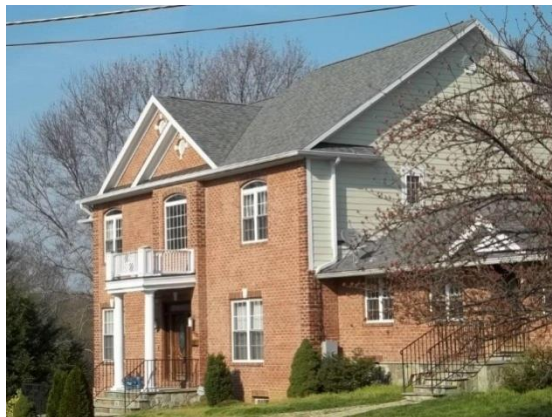
Figure 55: Firefighters should be aware of fire conditions above them in cross gable roofs.
