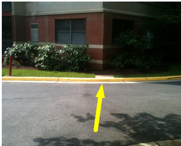
Figure 18: This photograph of an apparent sidewalk that terminates into a wall is actually a concrete pad placed at the corner of this high-rise building to provide support for a Truck's stabilizer.
