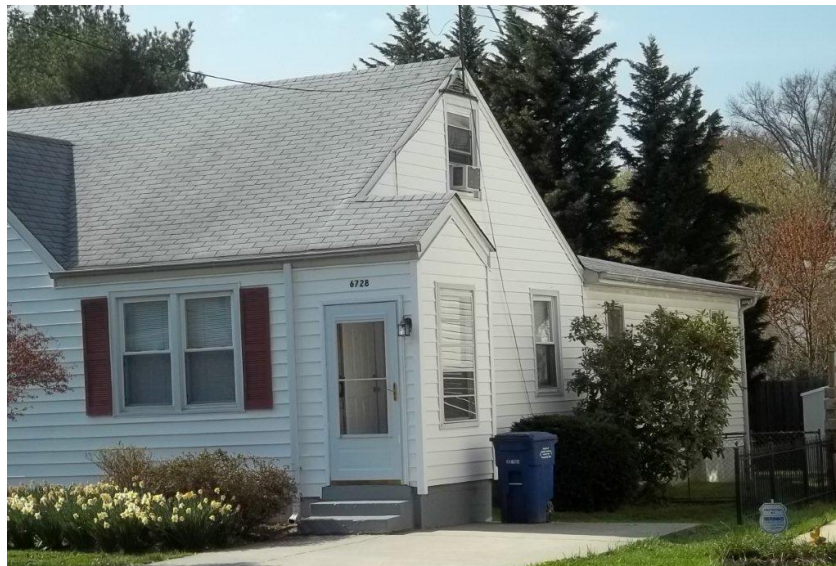
Figure 51: Cape Cod structure with an addition on the rear
