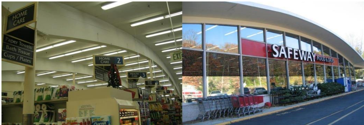
Figure 40: Laminated arch roof, common in old grocery stores.
