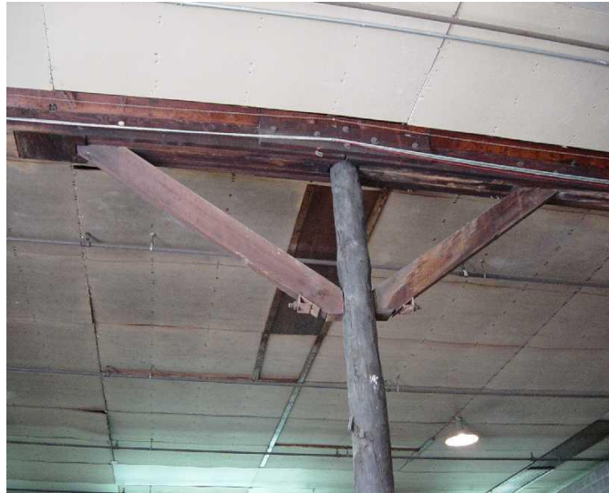
Figure 66: Column connector.
