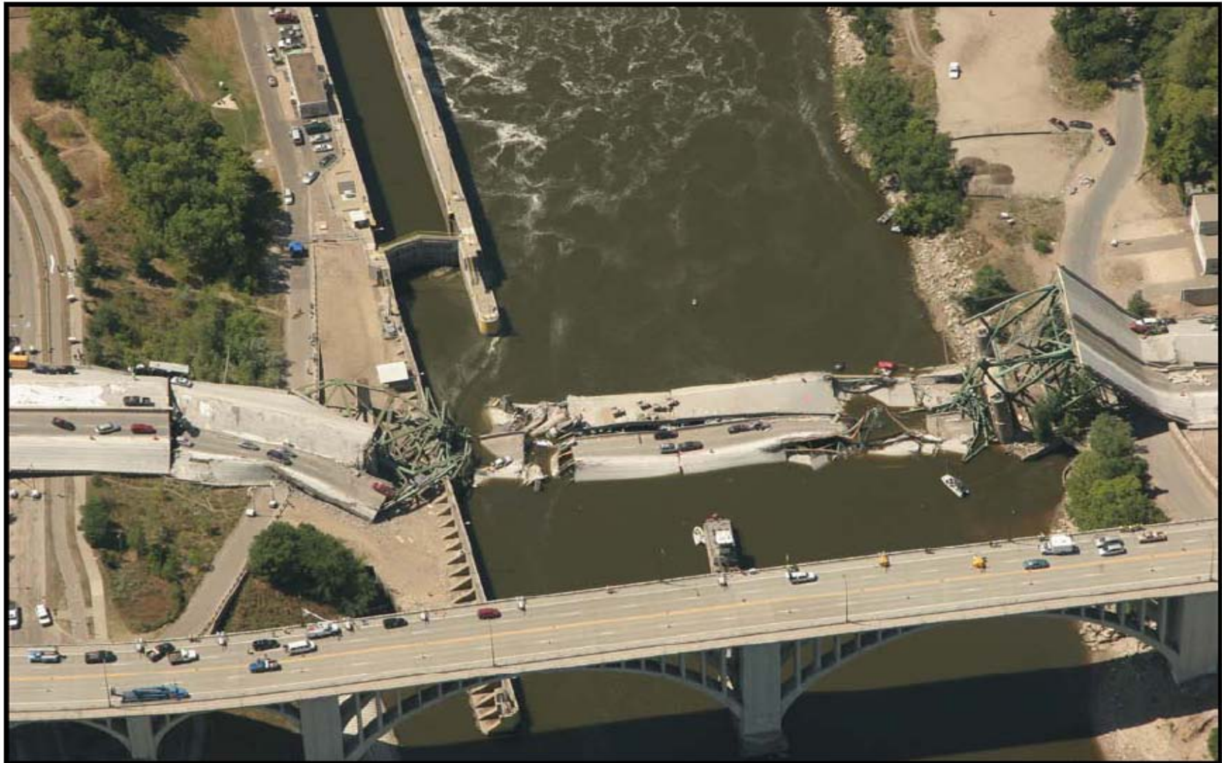
Post collapse, viewed looking west.
