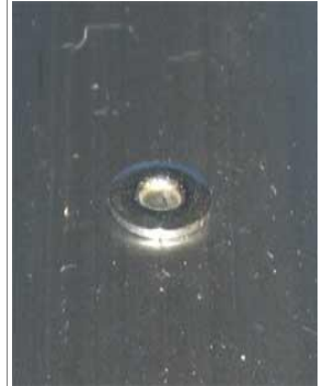
Outside hole with aluminum eyelet.
