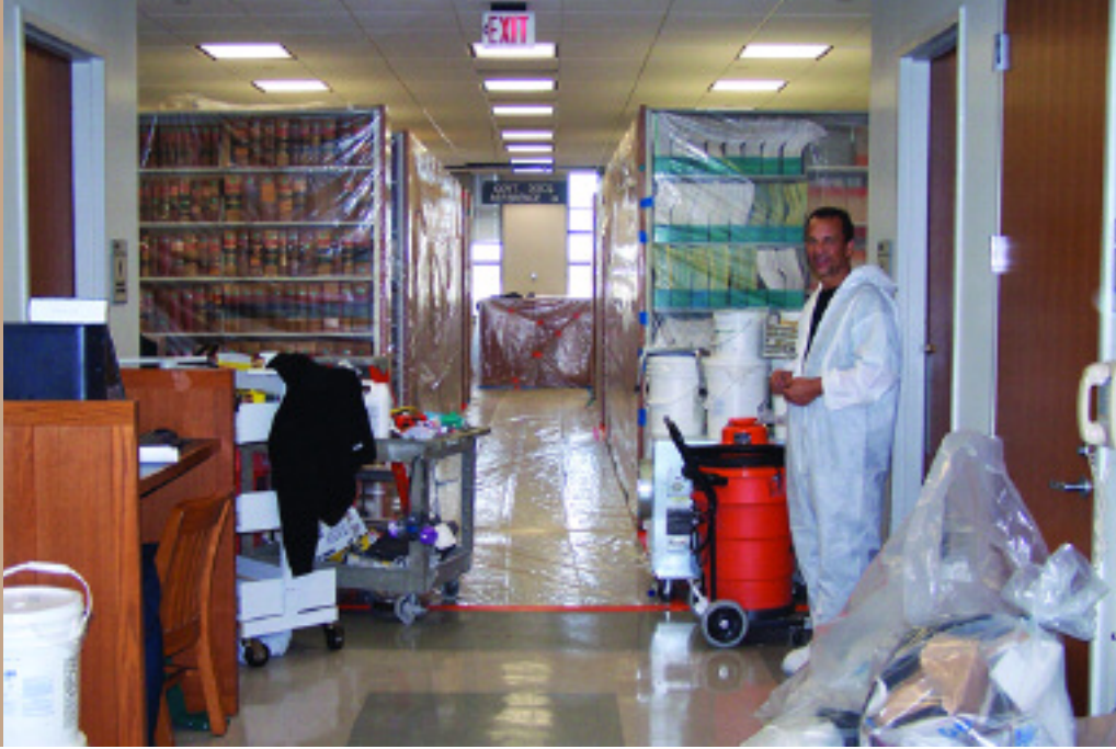
All six floors of Weinmann Hall including the Law Library underwent a thorough decontamination process after the storm. Photograph by Kim Glorioso.
